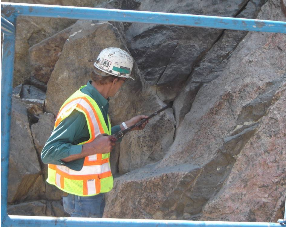
Figure 6. Photo. Insertion of the injection port/packer into drillhole.
