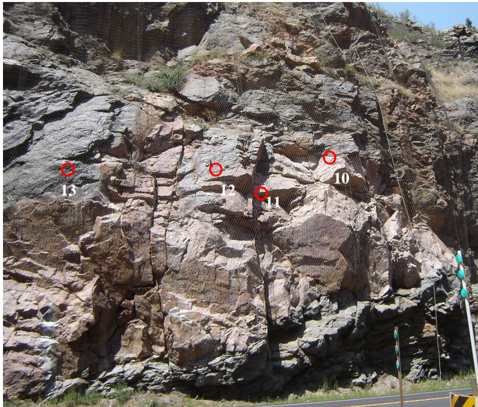
Figure 14. Photo. Approximate locations of selected PUR injection holes.
