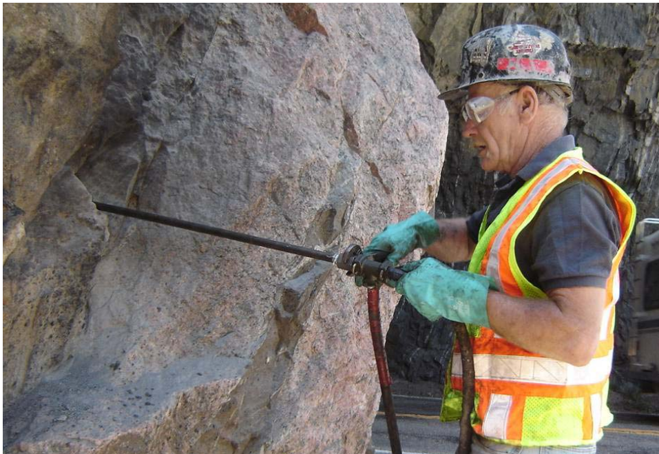
Figure 7. Photo. Connection of PUR Component A and B hoses to injection port.
