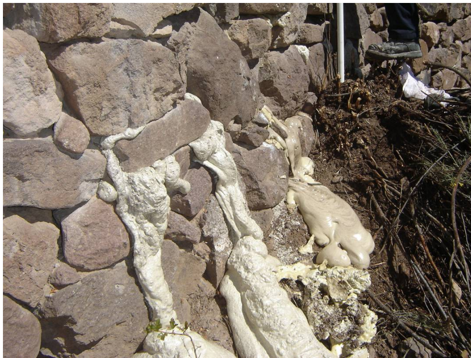
Figure 21. Photo. PUR that has foamed due to high moisture within the wall rock mass. This material can be readily peeled off the rock face and bagged for disposal.
