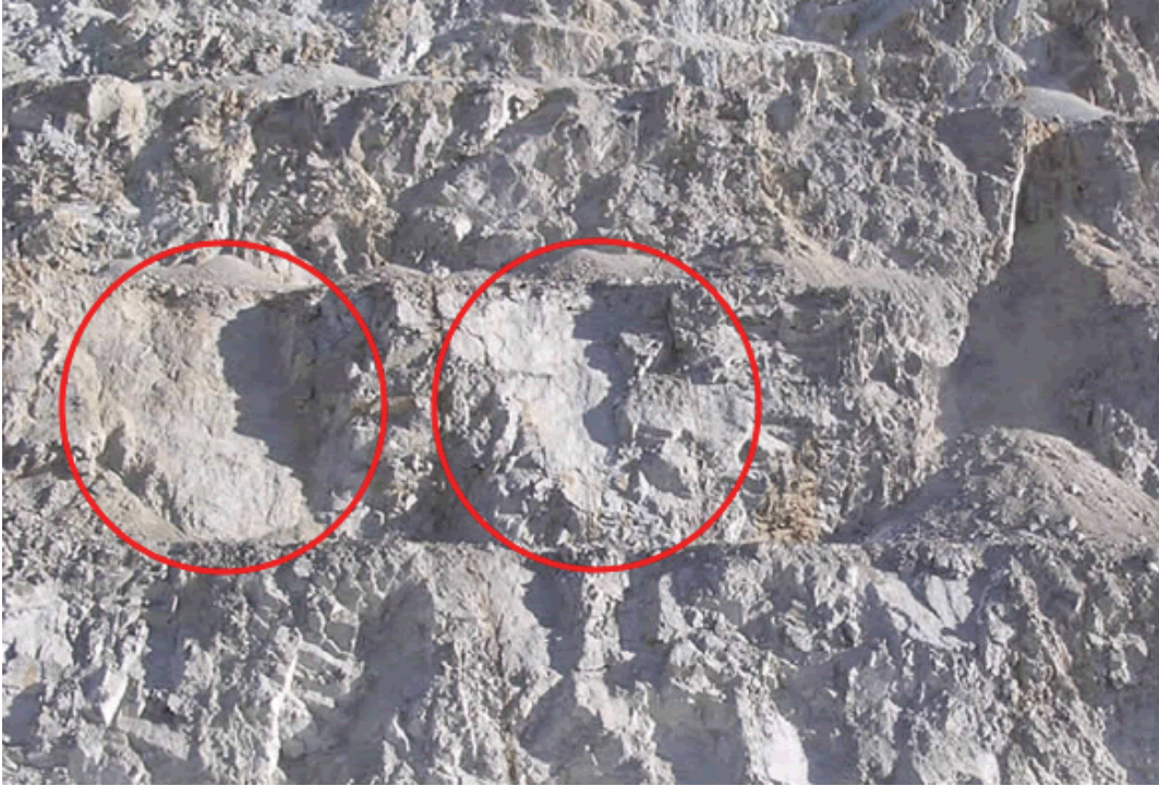
Figure 8a. Photo. Location of two large fractures for determination of maximum dilatation angle using the method described in Figure 7.
