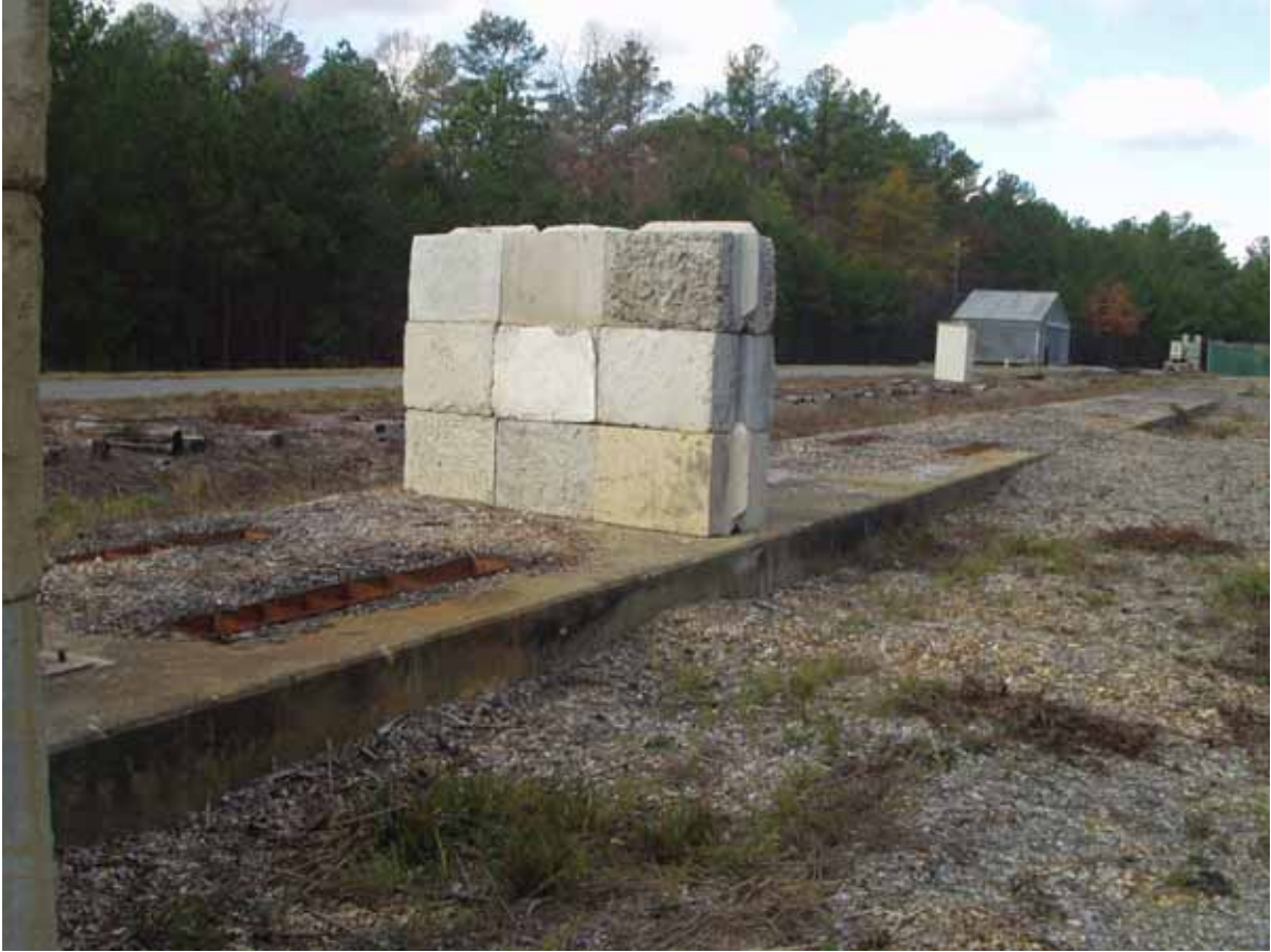
Item 5 looking west. Stacked gray blocks on the left and center are not associated with the Shock Tube. These concrete barriers are placed to prevent fragments from damaging nearby equipment. Visible in the background right of the picture are non-associated structures: upright white equipment shelter, gray building 1290A, and the green fence previously mentioned.
