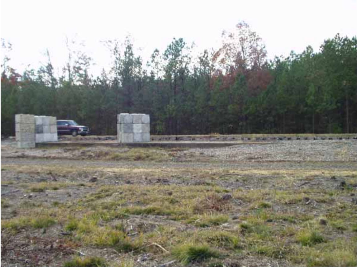
Looking south at the SE end of item 5. Stacked gray blocks on the left are not associated with the Shock Tube. These concrete barriers are placed to prevent fragments from damaging nearby equipment.
