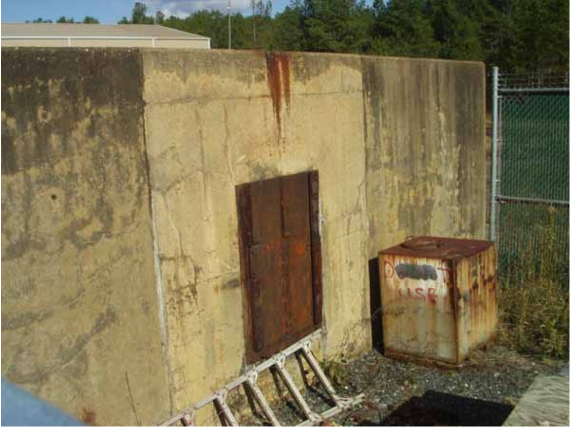
Item 1 thrust plate, Looking north.
