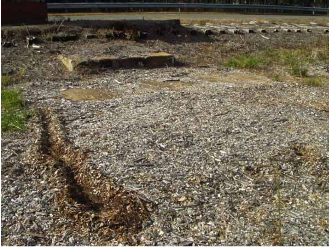
Looking west at items 16, a 4x7 slab stepping down to partially buried 16x16 slab. Shock Tube Road is in the background. The bottom of an equipment shelter is visible in the extreme upper left.
