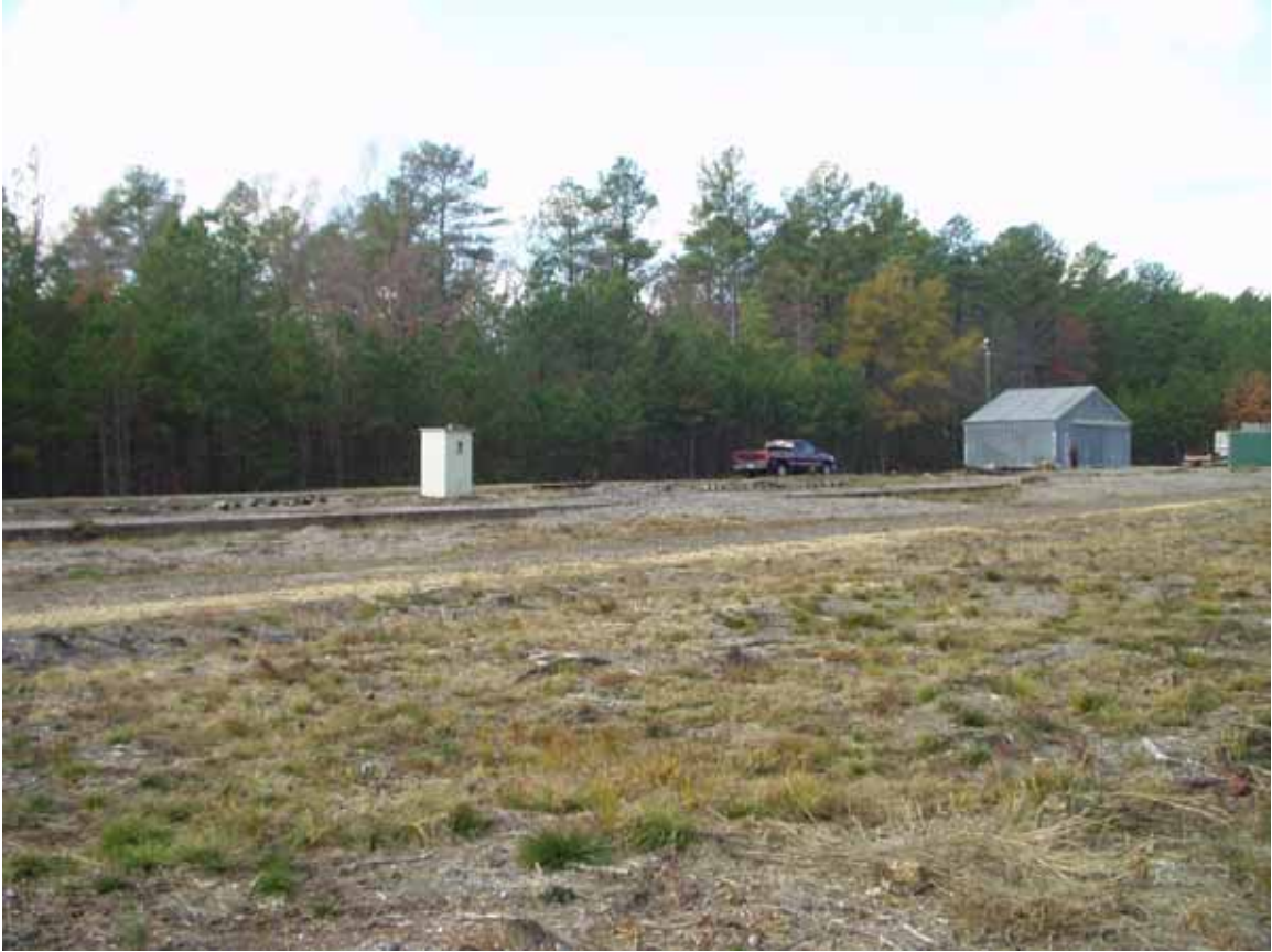
Looking west at the NW half of Item 5. Visible in the picture are non-associated structures: upright white equipment shelter, gray building 1290A, and green fence previously mentioned.
