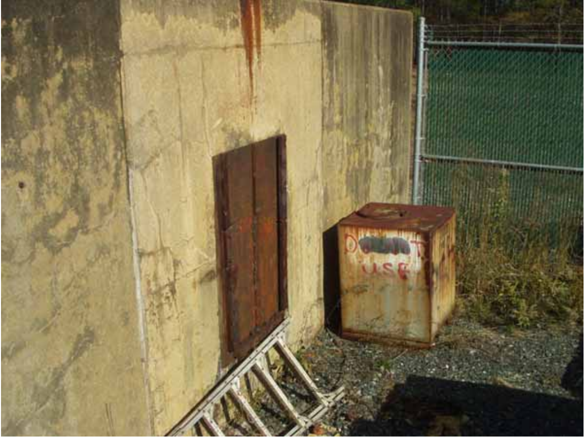
Item 1, Thrust plate, In Southeast end. Looking NNE.
