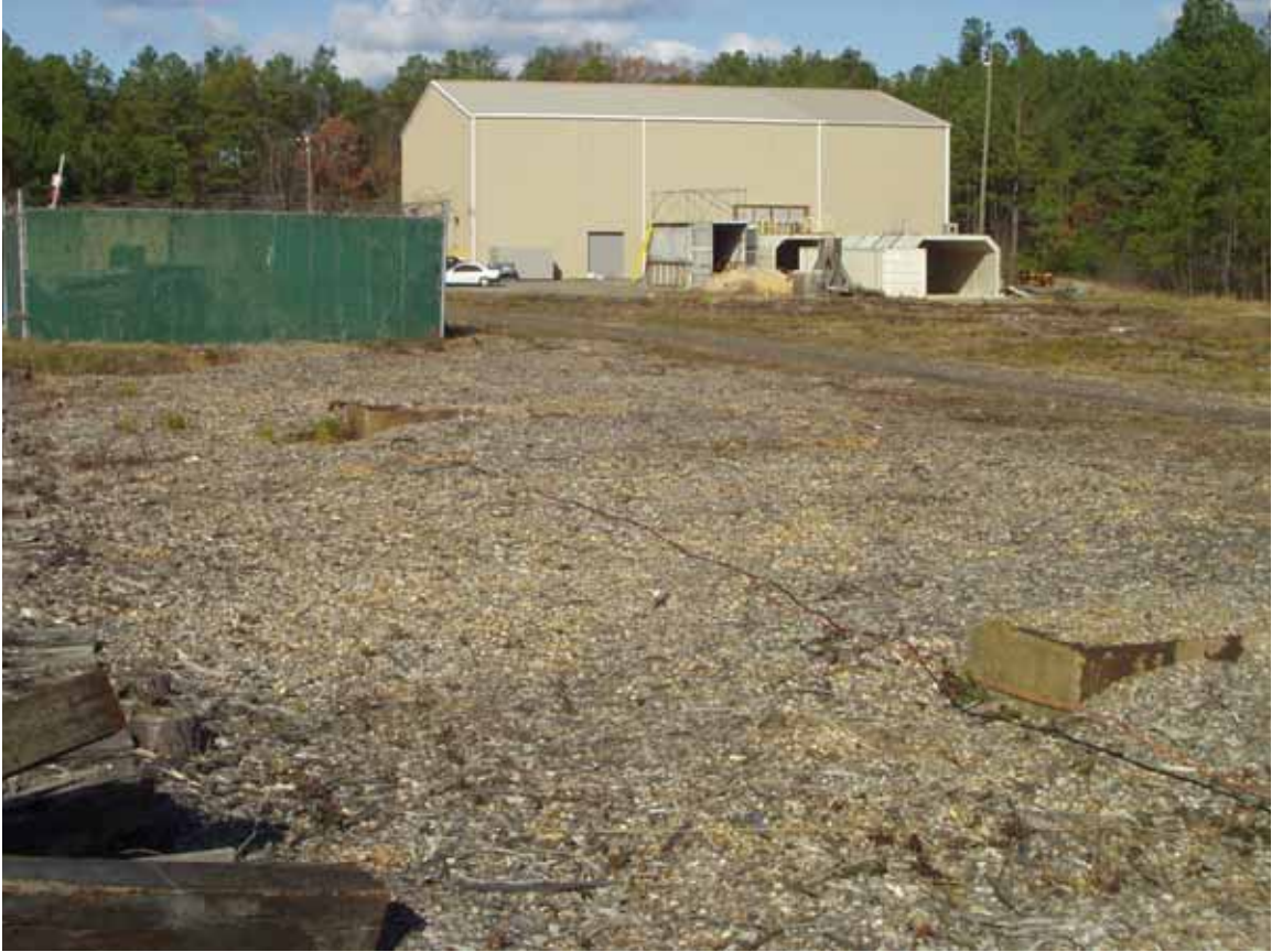
Items 2, 3, and 4; looking north. Item 4 is near right. Green fence and large tan building with associated structures in the background are not part of the Shock Tube.
