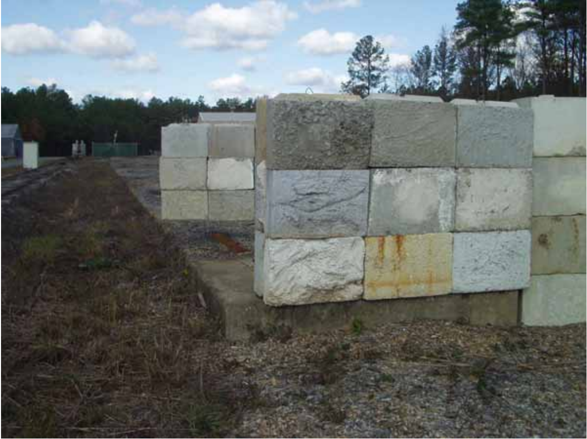
Item 5 looking north. Stacked gray blocks on the right and center are not associated with the Shock Tube. These concrete barriers are placed to prevent fragments from damaging nearby equipment. Visible in the background left of the picture are non-associated structures: upright white equipment shelter, gray building 1290A, and the green fence previously mentioned.
