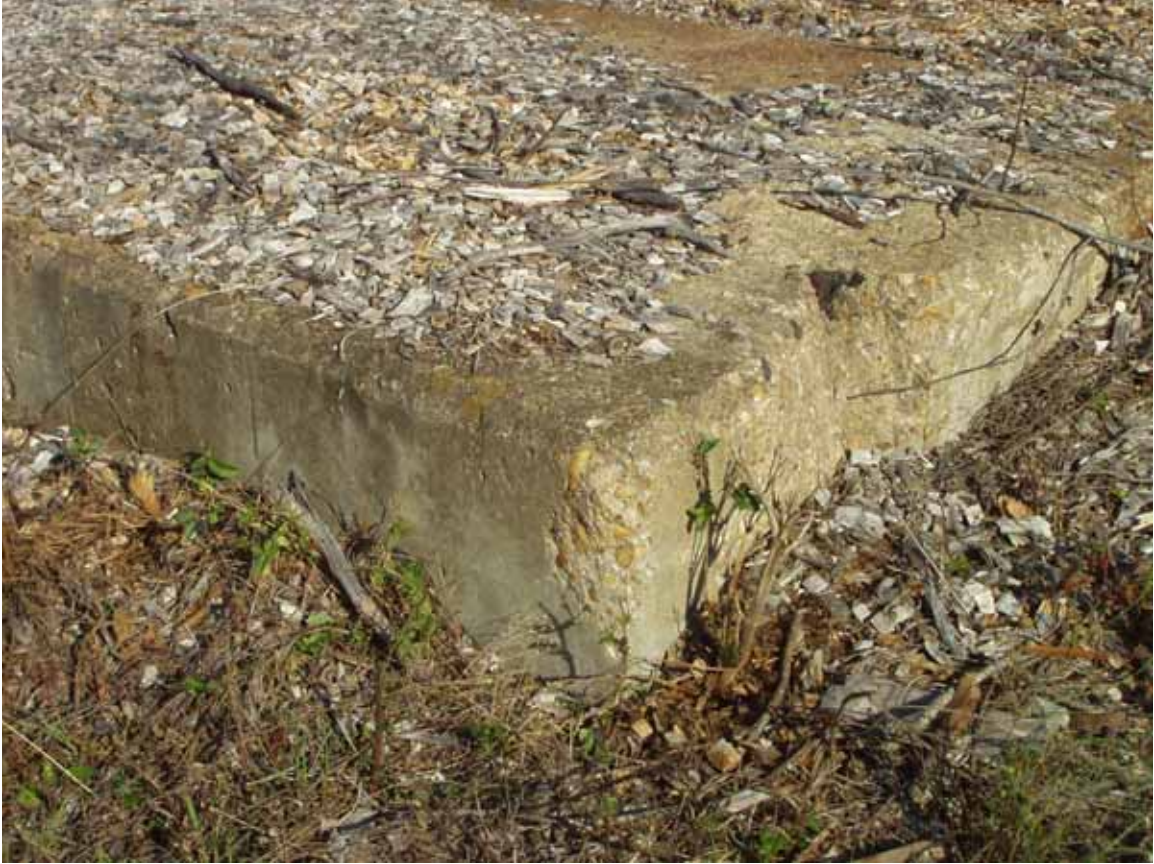
Item 24 showing typical construction of the pads.
