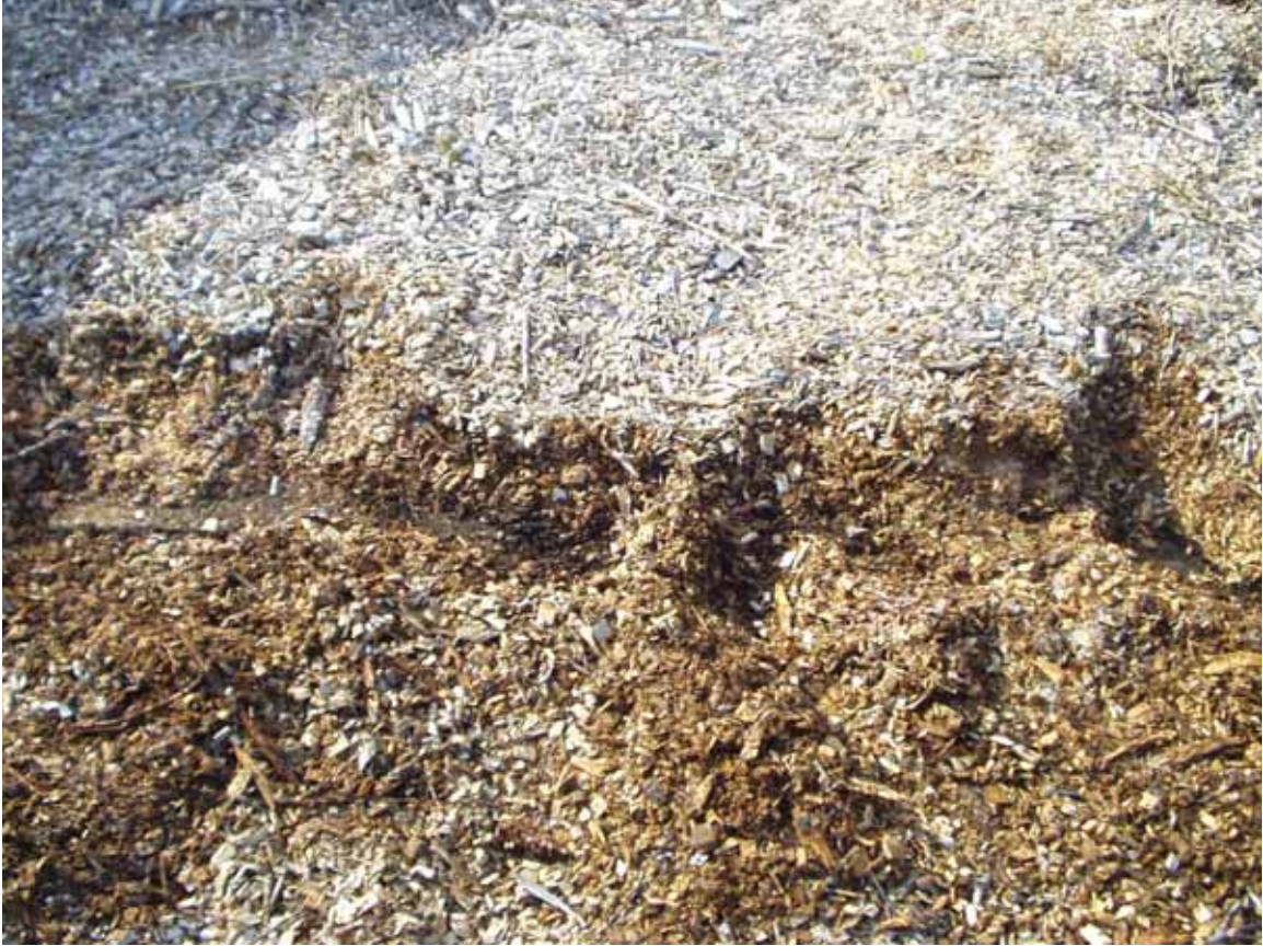
Item 6 is a smallish concrete pad whose dimensions are difficult to determine under heavy cover of wood chips.
