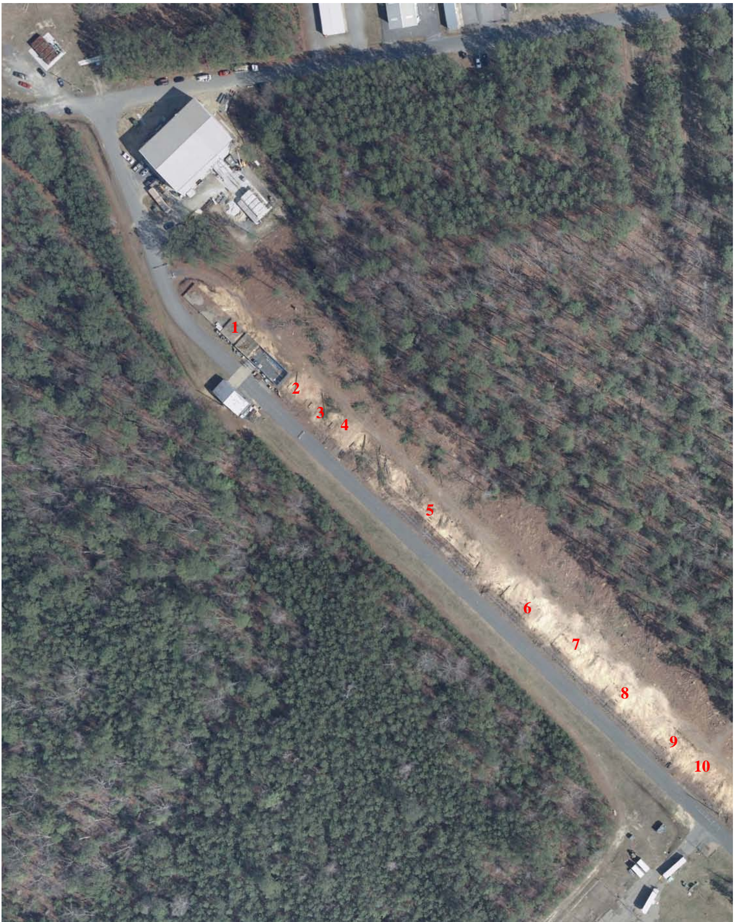
Conical Shock Tube Foundations After Removal Aerial Photography 2008 -- Overview of the North End, best viewed at 400% Numbers refer to items shown in detailed pictures taken 18 Nov 2008.
