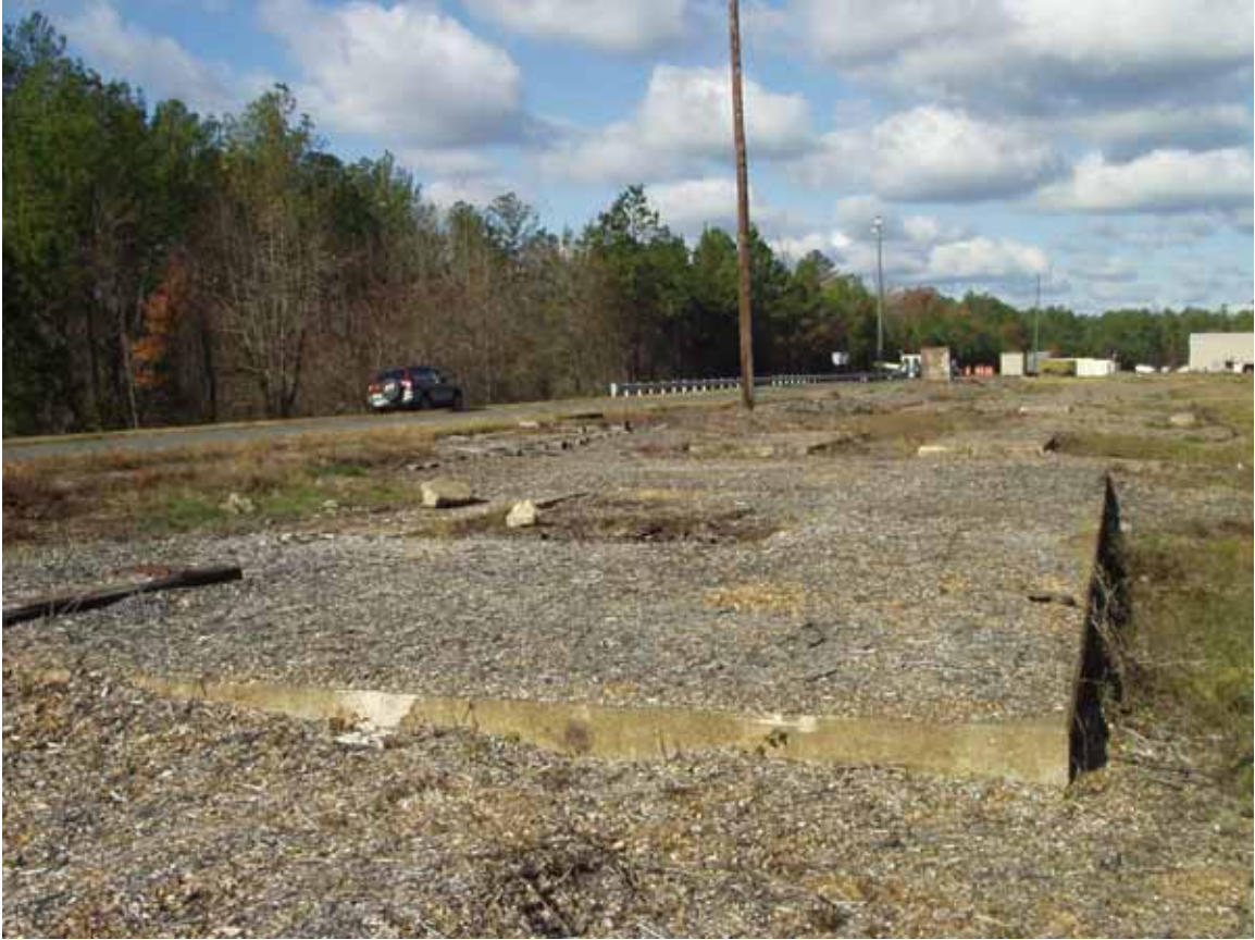
Looking NW at item 20, osprey nest pole is in the background.
