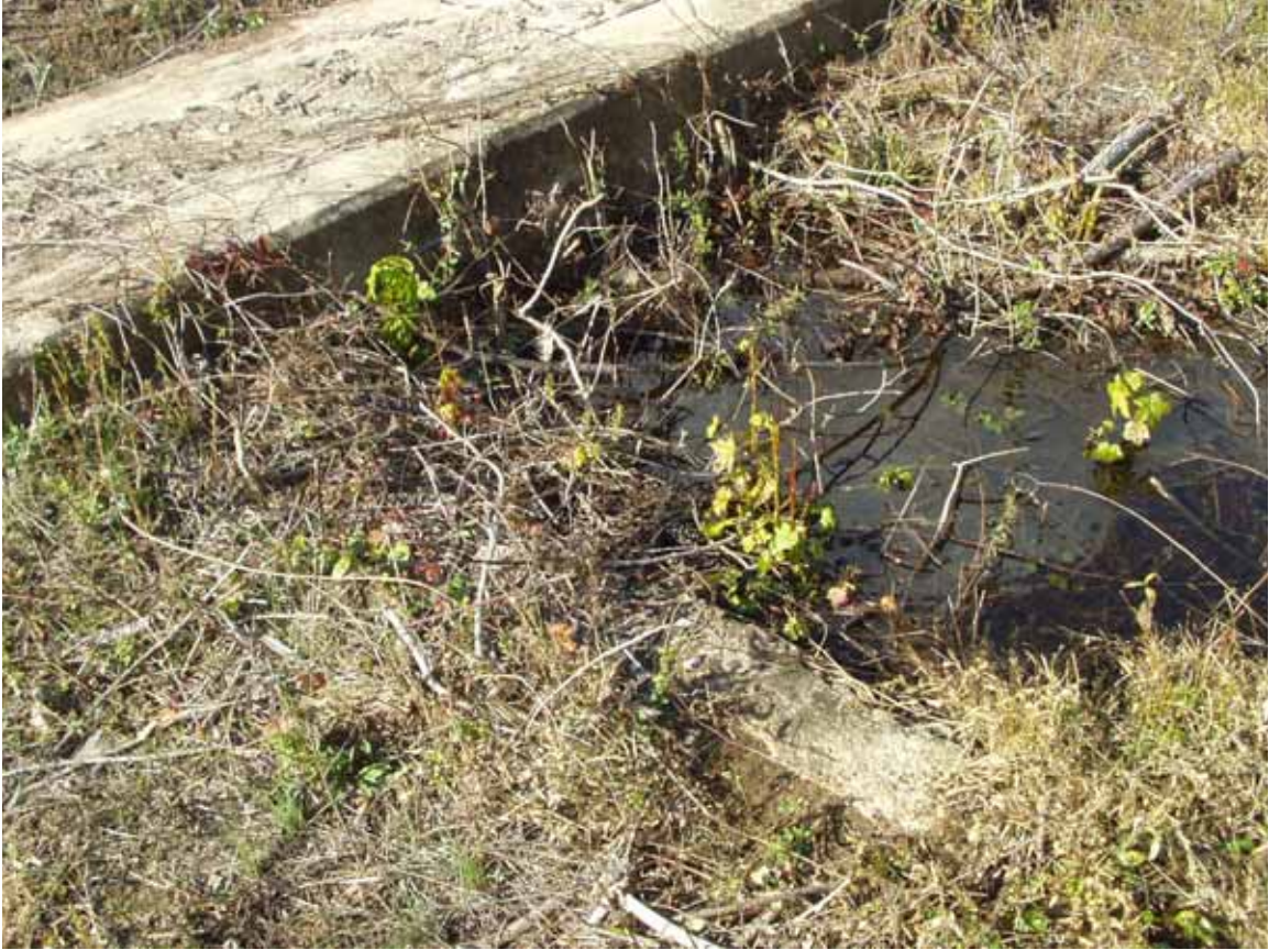
Item 23 has concrete beams tying the two separate 4x22 pads together.
