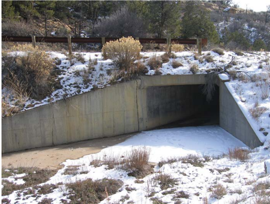
Figure 32. Photo. Cast-in-place concrete cantilever walls are commonly found serving as wingwall structures for large box culvert features within the WIP inventory.
