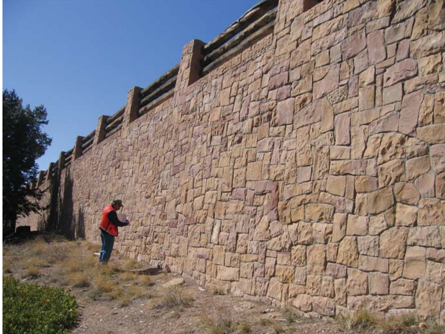
Figure 80. Photo. Although this stone masonry-faced MSE wall at Bryce Canyon National Park is a relatively new structure built to AASHTO standards, it is nonetheless culturally sensitive as it contributes to the cultural context of the roadway corridor.
