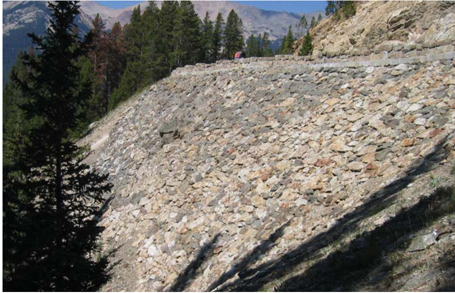
Figure 26. Photo. Machine- and hand-placed slope protection at Rocky Mountain National Park.
