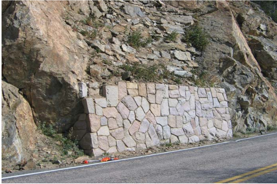
Figure 18. Photo. A mortared stone masonry cut wall at Rocky Mountain National Park.
