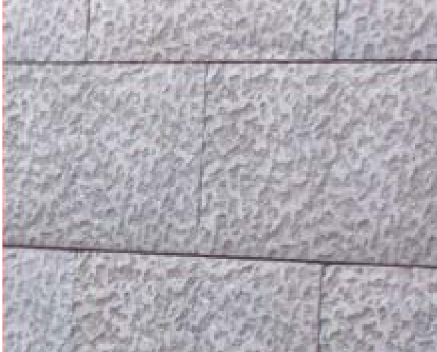
Figure 58. Photo. Example of concrete blocks textured with a bush hammer prior to placement. A range of textures can be created with this technique, depending on the hammer head size and configuration. (Courtesy Doublewal Corporation)
