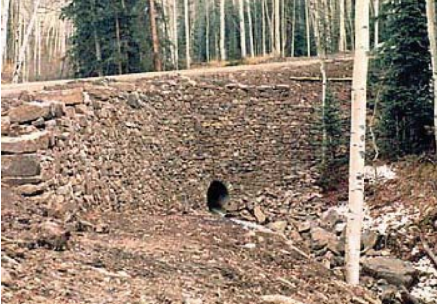
Figure 55. Photo. Single-course, mortared stone facing placed in front of an MSE wall structure. Well-built facings can make it very difficult to discern modern facades from historical structures. (Courtesy Mountain Village Metropolitan District, Telluride, CO)
