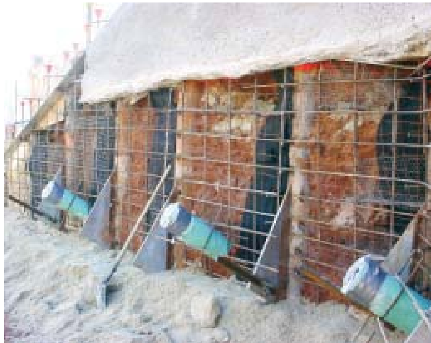
Figure 28. Photo. Micropile tieback wall prior to shotcrete facing finish (ADSC, 2006).
