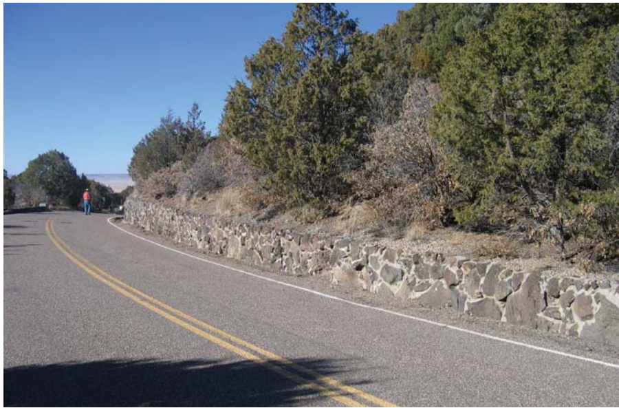
Figure 11. Photo. This culturally sensitive, mortared stone masonry cut wall at Capulin Volcano National Monument falls under the height requirement over the majority of its ~300 ft length, with only a short section extending above the minimum 4 ft acceptance criterion. Should the entire wall be included in the inventory? (Yes, per the discussion provided later in this section.)
