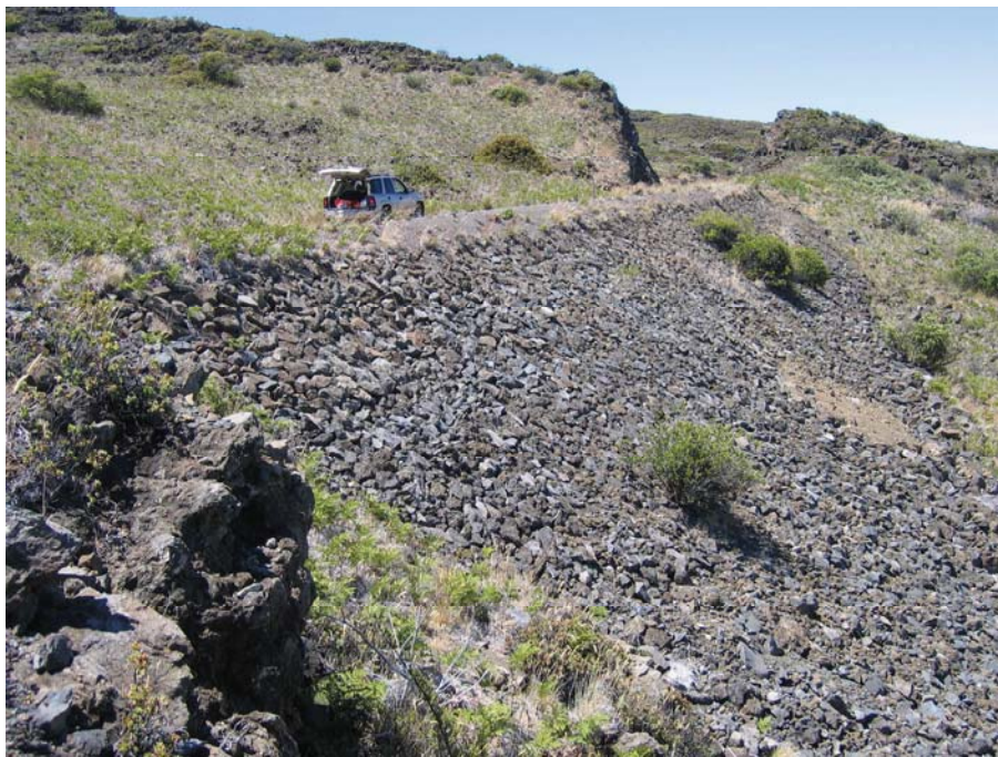
Figure 13. Photo. This placed stone retaining structure, with a 50^{\circ} face angle, retains the fill slope supporting the roadway at Haleakala National Park and could be included in the WIP.
