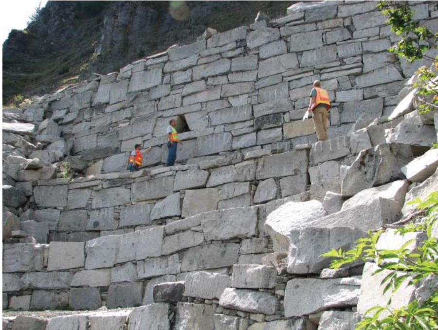
Figure 9. Photo. Inventory team members must work together to measure wall attributes, accurately describe and rate wall elements, and watch for unsafe conditions.
