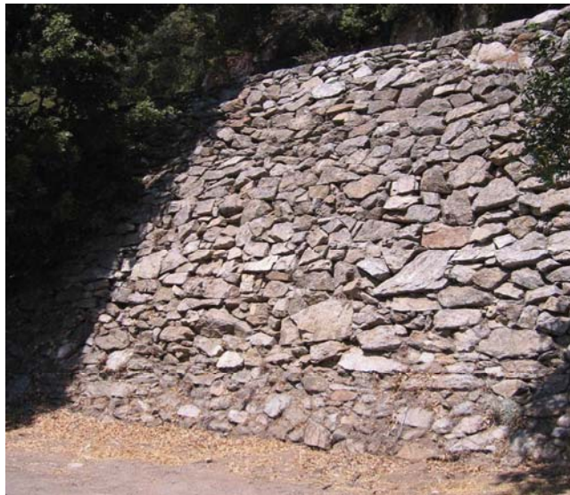
Figure 24. Photo. Example of a mortared stone masonry switchback wall at Sequoia National Park between upper and lower roadway on the inside of a switchback curve.
