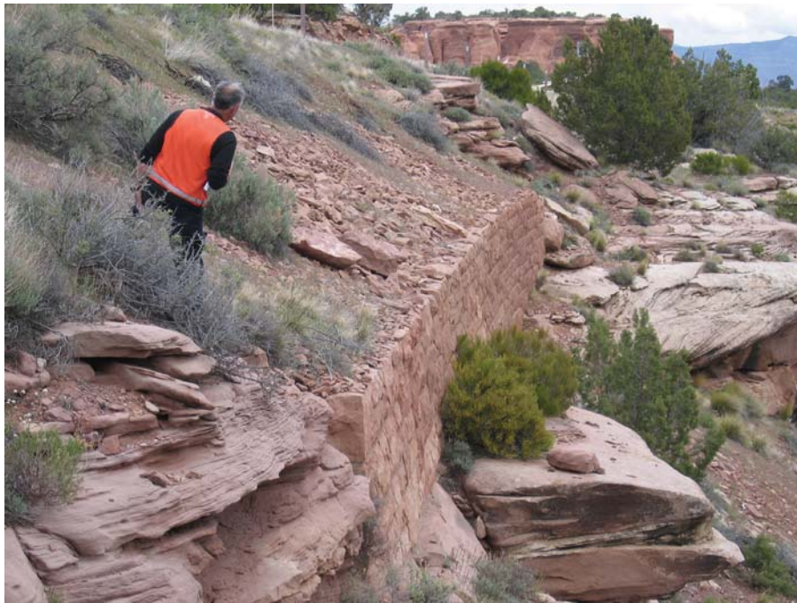
Figure 15. Photo. Retaining walls are found in a wide array of settings. Wall performance is impacted by factors other than constructed components, including foundation materials, top and side slopes, vegetation, drainage, etc.
