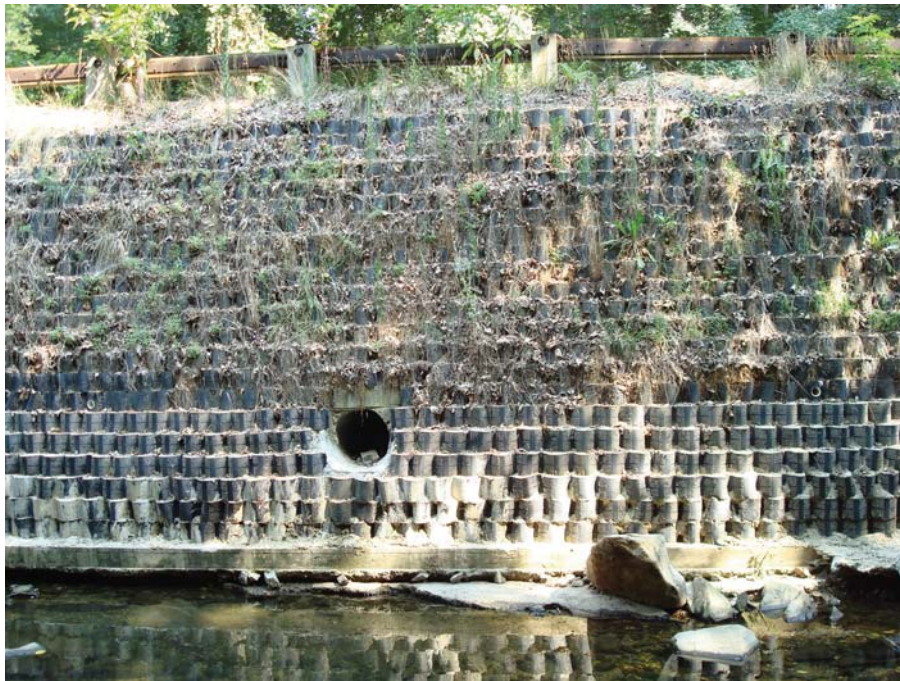
Figure 49. Photo. “Other” wall type: geosynthetic reinforced earth wall with planted geocell facing. This wall facing method may prove to be a superior means for establishing face vegetation in high growth climates. Note the installation of the concrete leveling pad.
