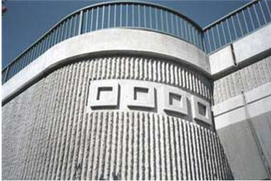
Figure 51. Photo. Example of one of the many “Fractured Fin” formliner architectural facing treatments available and commonly used in urban construction. (Courtesy Fitzgerald Formliners)
