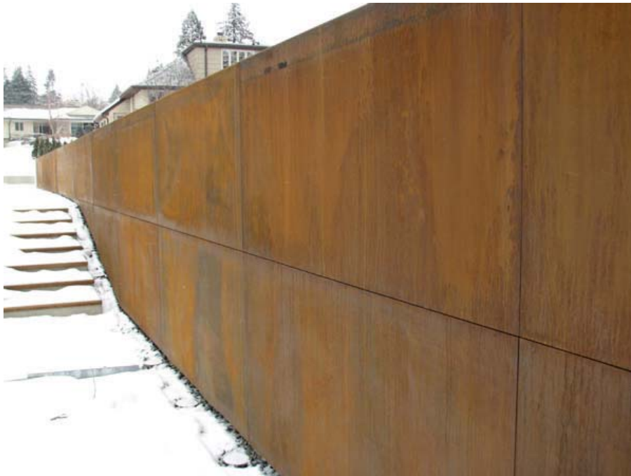
Figure 62. Photo. Weathering steel, sold under the “CORTEN” trademark, can provide a long-life, low-maintenance surface treatment for wall systems in the right environment. (Courtesy Richer Metal, Dodge Center, MN)
