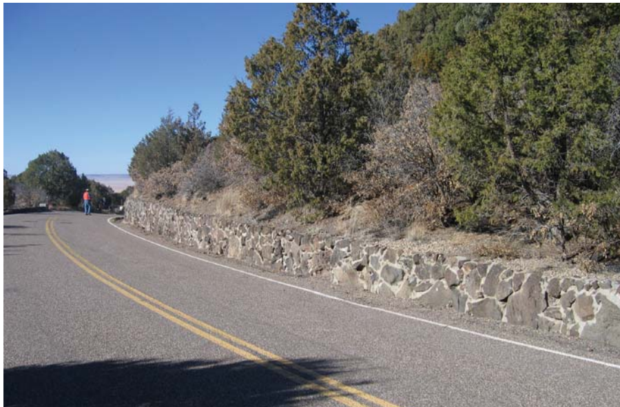
Figure 11. Photo. This culturally sensitive, mortared stone masonry cut wall at Capulin Volcano National Monument falls under the height requirement over the majority of its ~300 ft length, with only a short section extending above the minimum 4 ft acceptance criterion. Should the entire wall be included in the inventory? (Yes, per the discussion provided later in this section.)
