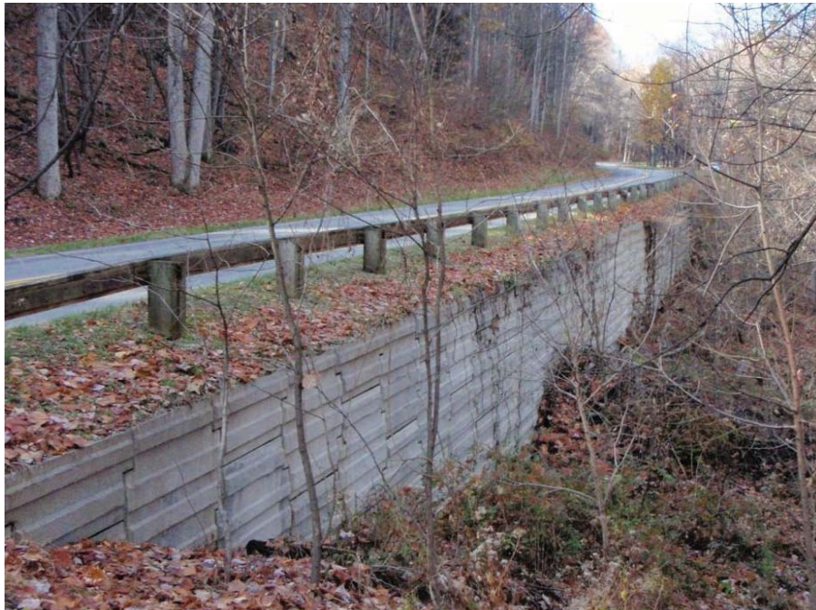
Figure 44. Photo. Precast panel MSE wall at Great Smoky Mountains National Park. A variety of architectural facing options are available, including formed concrete and stained or painted treatments.
