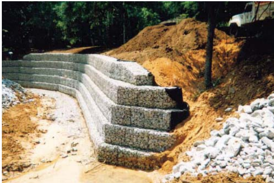
Figure 17. Photo. A gabion gravity fill wall under construction below roadway grade.
