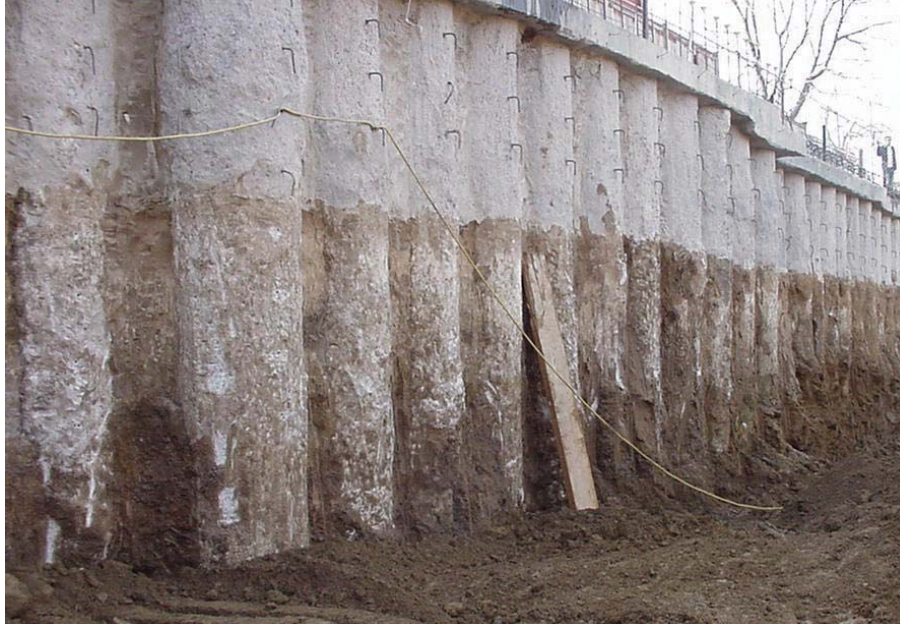
Figure 48. Photo. Tangent pile cut wall constructed of drilled shafts. This expensive wall system is primarily used where top-down soil nail or ground anchor construction is not feasible due to subsurface obstructions within the retained ground mass.
