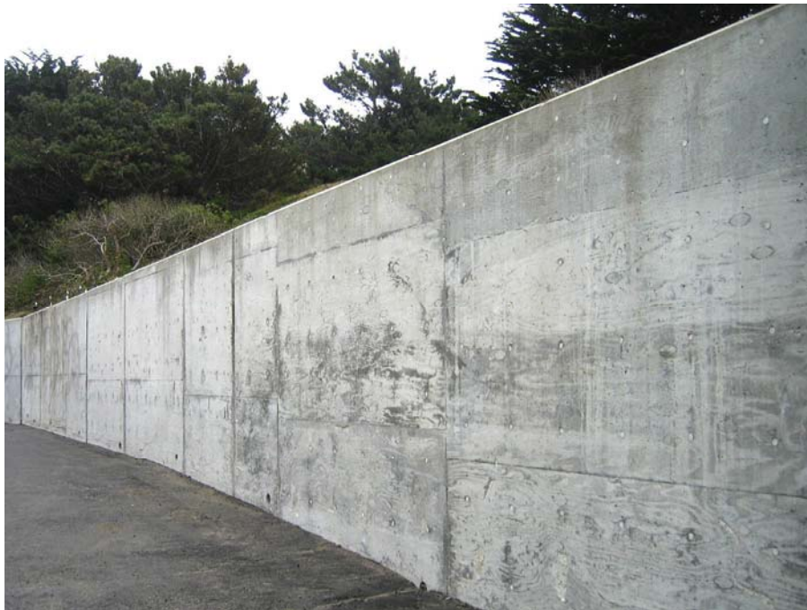
Figure 52. Photo. Although a seemingly accidental wall finish, a rough wood formliner was actually used in the construction of this concrete cantilever wall at Golden Gate National Recreation Area to simulate historical concrete construction practices throughout the park. This example emphasizes the need to discuss the cultural attributes of retaining walls with park resource staff prior to undertaking site inspections.
