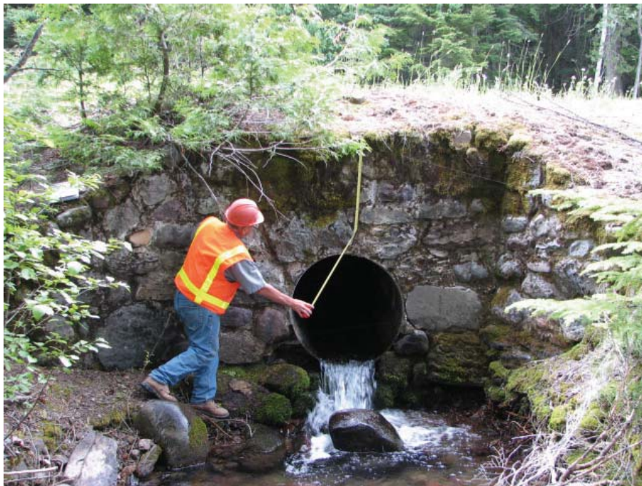
Figure 12. Photo. This outlet headwall and adjacent wingwalls clearly meets the culvert height criterion and directly supports the overlying roadway.
