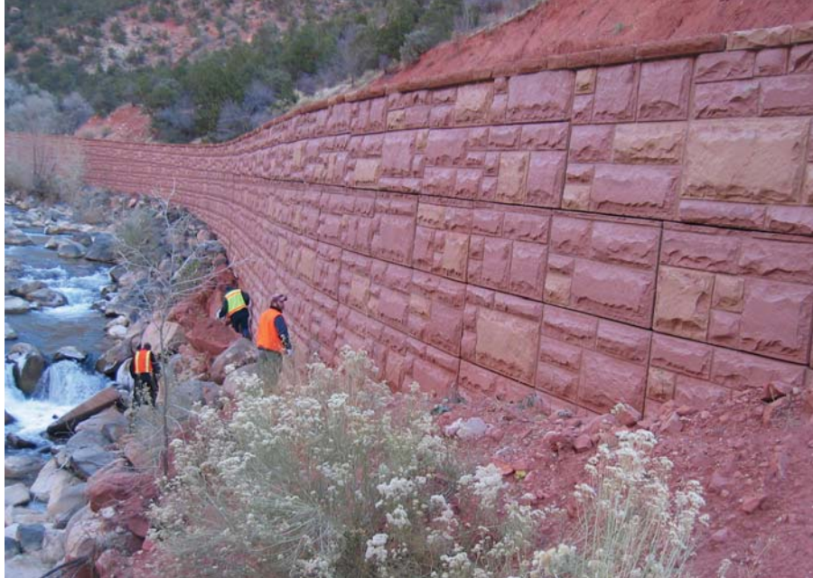
Figure 50. Photo. “Other” wall type: segmental concrete “T” wall at Zion National Park. Each precast “T” panel has concrete ribs extending into the compacted retained fill to serve as ground reinforcement and facing panel anchorage. The Ashlar block formliner was stained to match the surrounding country rock.
