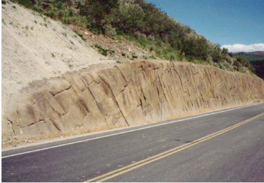
Figure 61. Photo. Example of sculpted shotcrete stained to match the surrounding landscape. Fading due to seasonal weathering and UV damage may require additional staining to meet aesthetics objectives.
