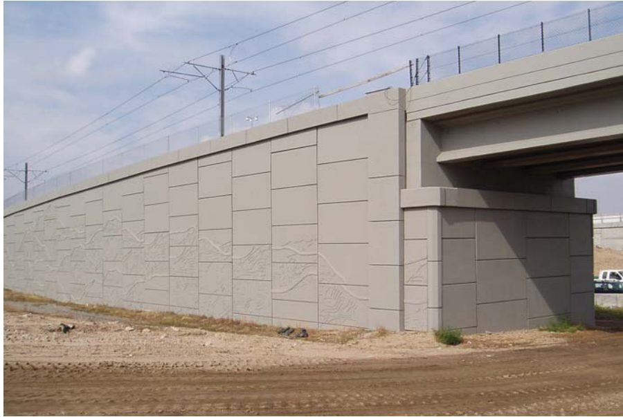
Figure 20. Photo. Although the approach walls are integral to the bridge abutment, they extend sufficiently from the end of the deck to be considered fill walls primarily supporting the roadway. Approach walls such as these should be included in the WIP inventory if not already evaluated under the BIP program.
