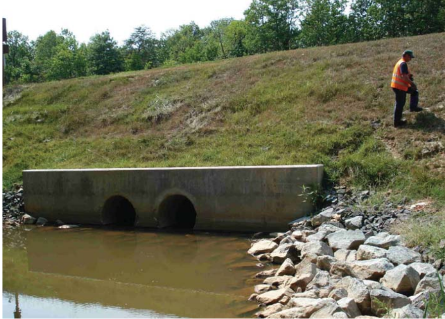
Figure 72. Photo. Assuming the head wall height meets the 6-ft criterion, the overlying slope would be evaluated as an “Upslope” secondary element.
