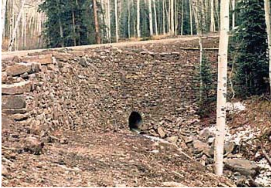
Figure 55. Photo. Single-course, mortared stone facing placed in front of an MSE wall structure. Well-built facings can make it very difficult to discern modern facades from historical structures. (Courtesy Mountain Village Metropolitan District, Telluride, CO)
