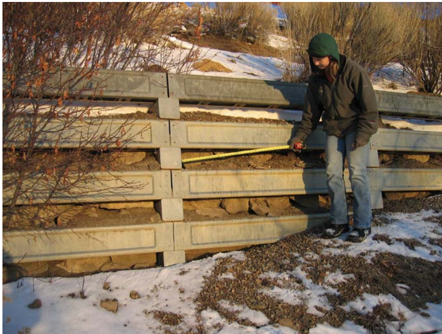
Figure 36. Photo. Metal crib wall at Mesa Verde National Park. Large rock fill was used on this wall to avoid the need for facing mats to retain fill aggregate.
