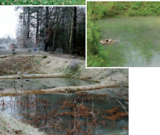
Subsurface gravel wetlands do an exceptional job of treating stormwater quality and managing water quantity. The design for the gravel wetland pictured above is helping New Hampshire's Department of Transportation meet Total Maximum Daily Load (TMDL) standards for numerous transportation improvement projects.
