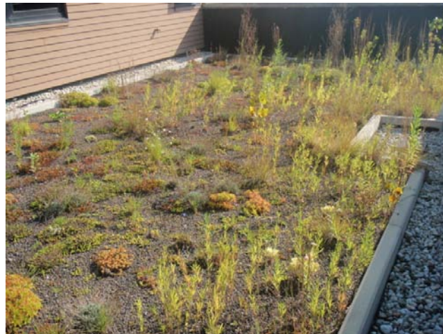
10 11 Figure 10: Villa Park Police Station Green Roof 62
