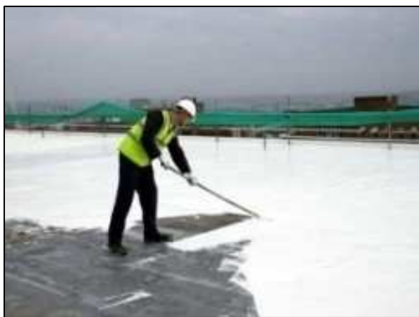
Figure 3: Creating a white roof is relatively simple
