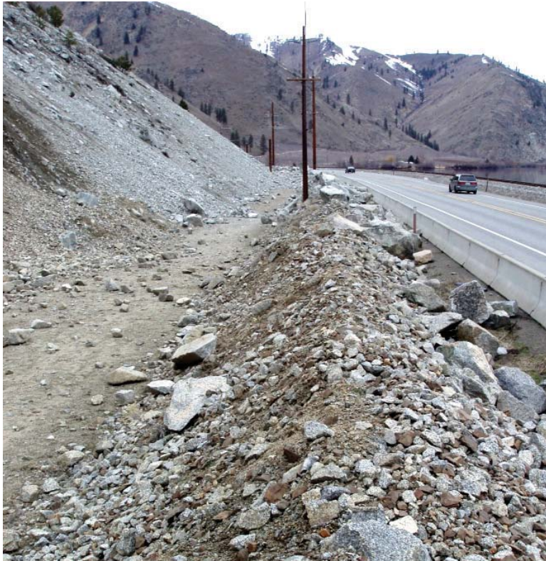
Figure 65. Photo. A conventional earthen berm can protect a highway from rockfall with low bounce height and low rotational energy.
