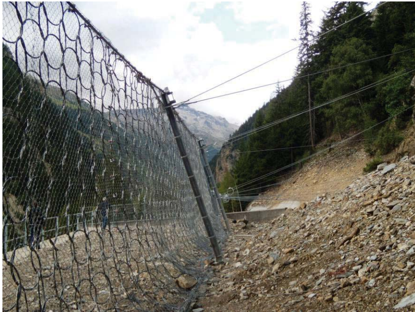
Figure 68. Photo. Example of a ring-net flexible barrier.
