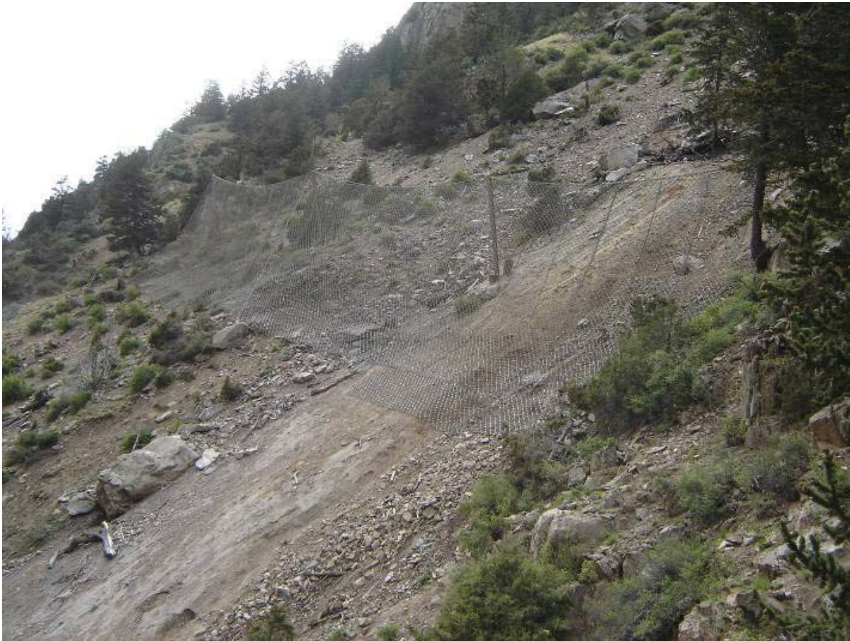
Figure 70. Photo. An attenuator combines a standard fence with a draping system. Georgetown, Colorado.
