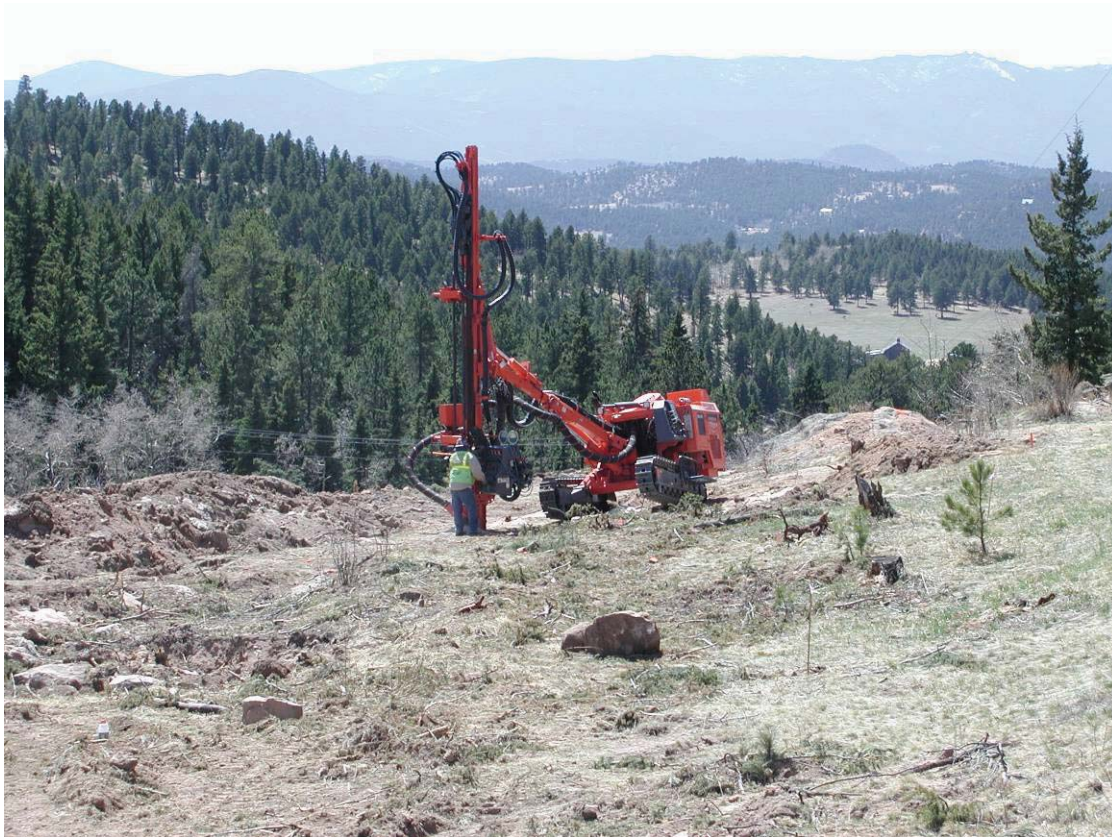
Figure 19. Photo. Common track drill used to advance vertical blastholes.
