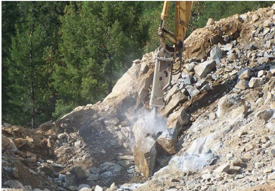
Figure 23. Photo. Application of a hydraulic hammer attached to an excavator.
