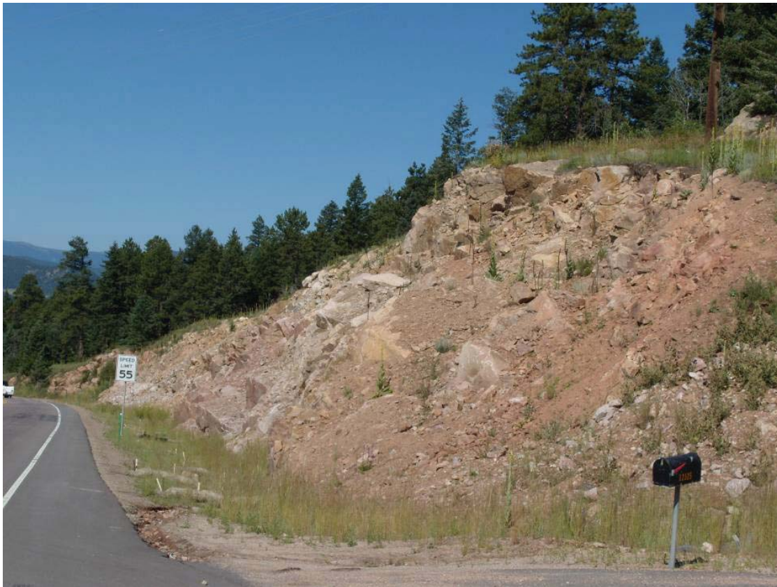
Figure 14. Photo. Final configuration of a cushion-blasted slope in granitic rock.
