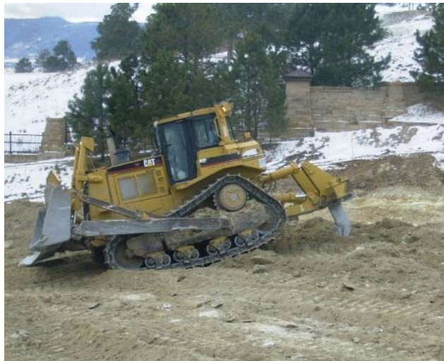
Figure 21. Photo. Bulldozer with an integral ripping attachment.
