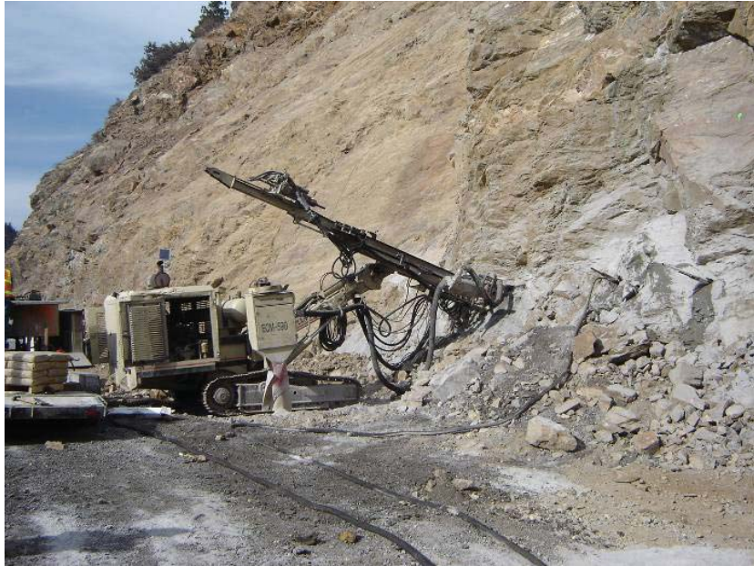
Figure 46. Photo. Installation of rock bolts using a track drill.
