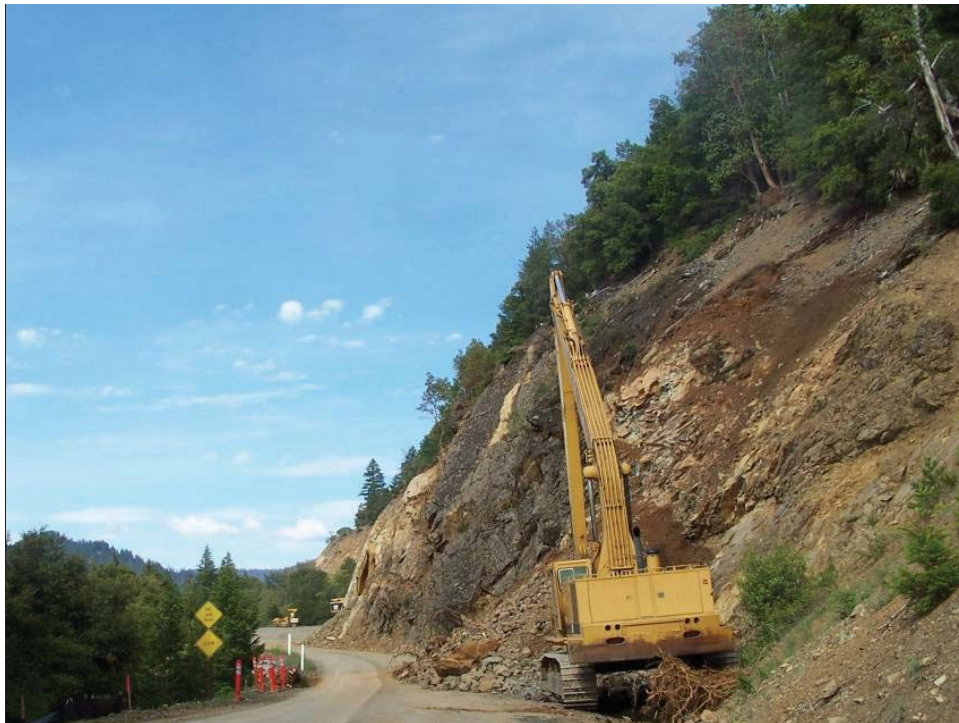
Figure 28. Photo. Slope rounding using long-reach excavator, Hyampom Road, California.
