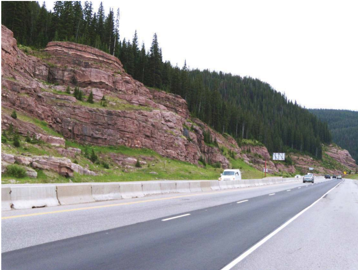
Figure 34. Photo. Steep, exposed rock faces are good candidates for slope angle variations.
