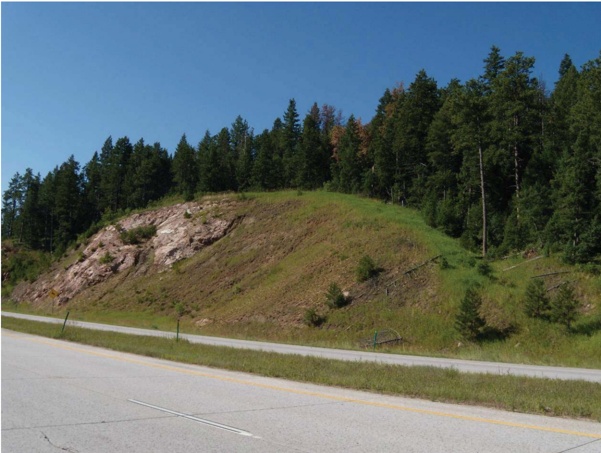
Figure 27. Photo. Example of major slope warping on a cut slope.
