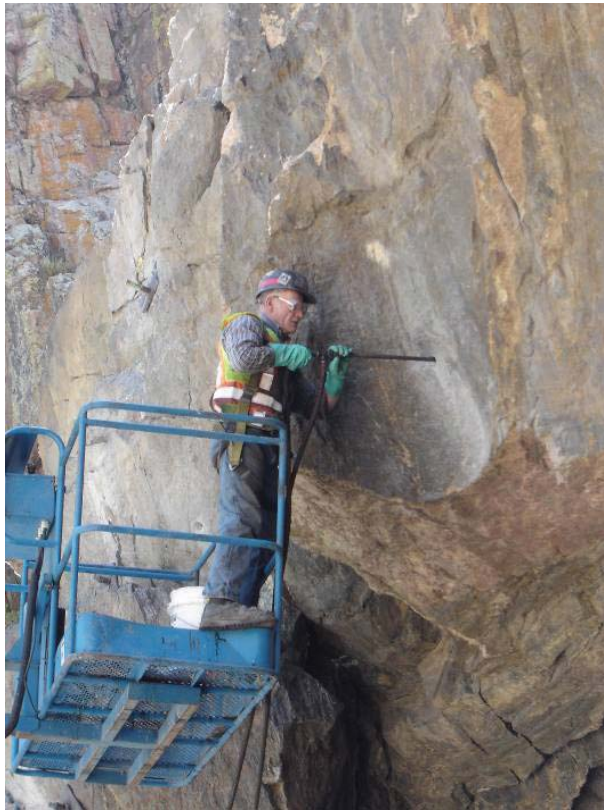
Figure 48. Photo. Installation of polyurethane resin from man lift, Poudre Canyon, Colorado.
