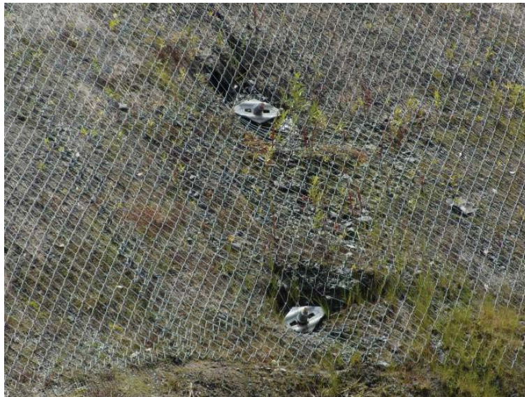
Figure 63. Photo. A detail of the anchors used to secure the mesh system shown above.
