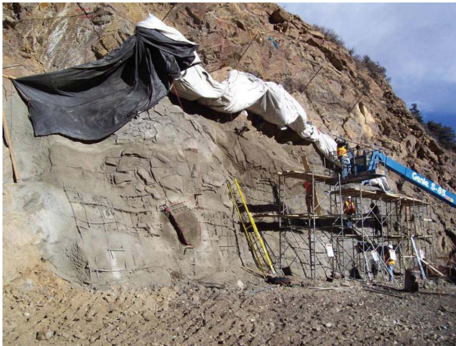
Figure 55. Photo. Application of the final sculpted shotcrete façade.
