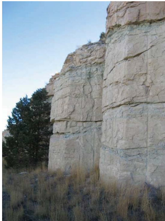
Figure 31. Photo. Ditch width variation used to break up the slope face and mask drill hole traces.
