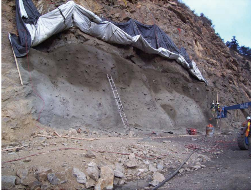
Figure 54. Photo. Installation of the first layer of structural shotcrete.
