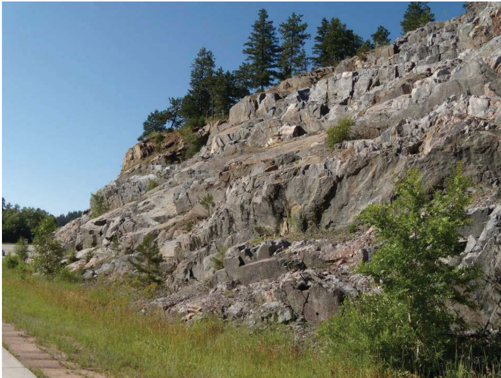
Figure 35. Photo. Rock slope excavated using slope variation and sculpting techniques.
