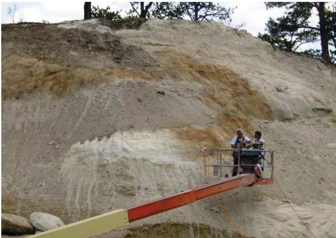
Figure 38. Photo. Application of stain to a newly constructed rock slope.
