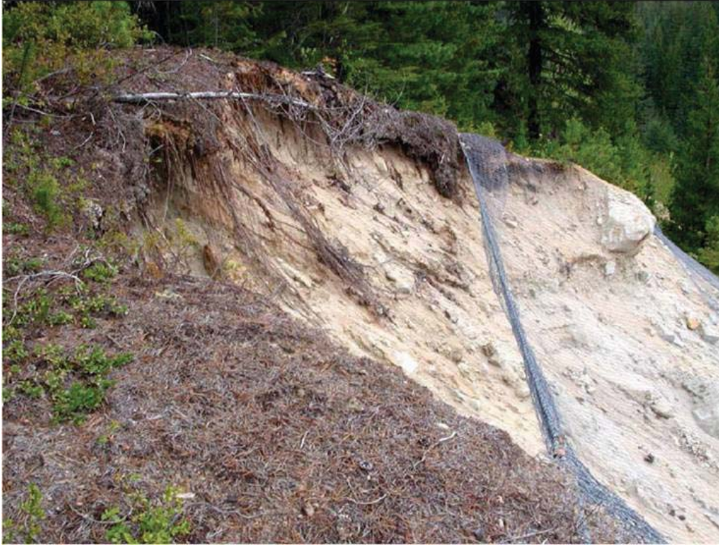
Figure 59. Photo. Erosion can lead to failure in a drapery system if the mesh is not secured sufficiently beyond the area of slope degradation at the top of the slope.
