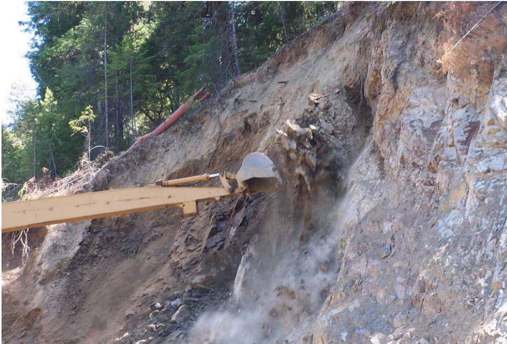
Figure 40. Photo. Using a long-reach excavator for mechanical scaling.
