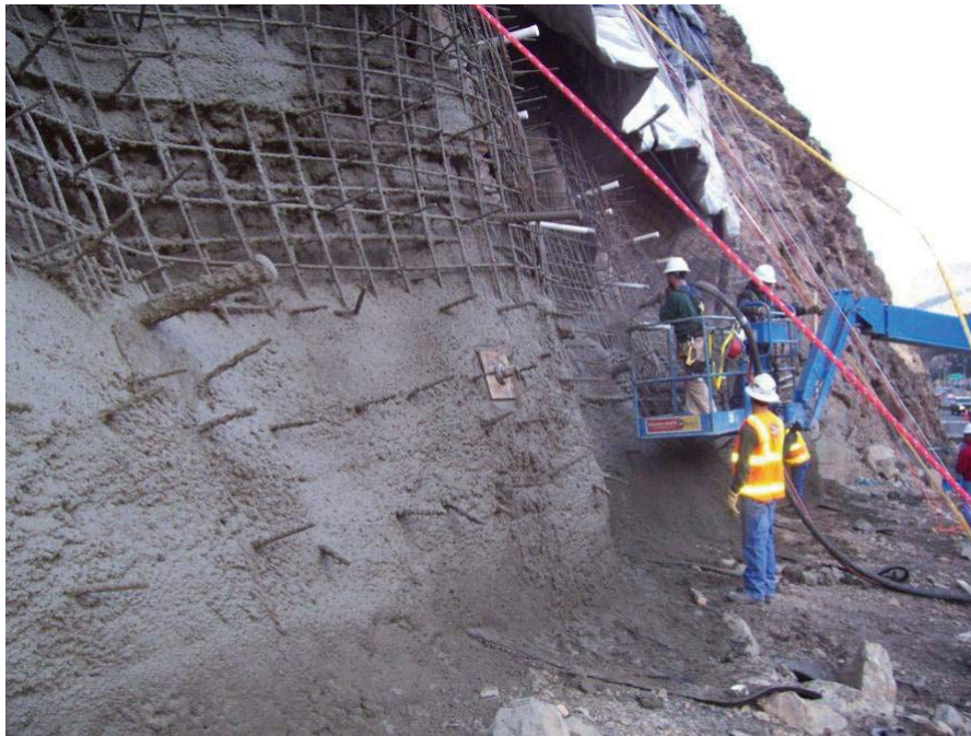
Figure 53. Photo. Application of the first layer of structural shotcrete.
