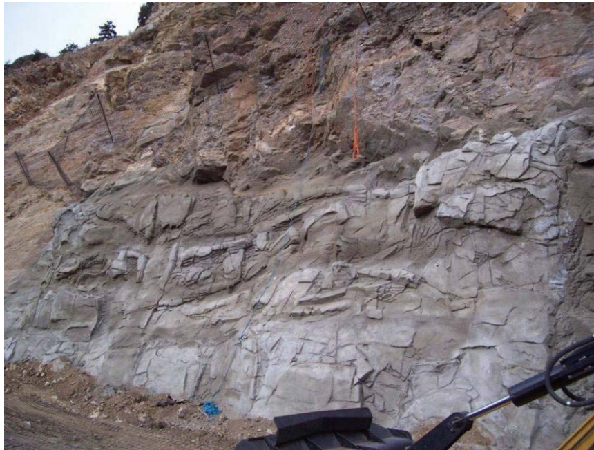
Figure 56. Photo. Completed structural shotcrete support, ready for staining.
