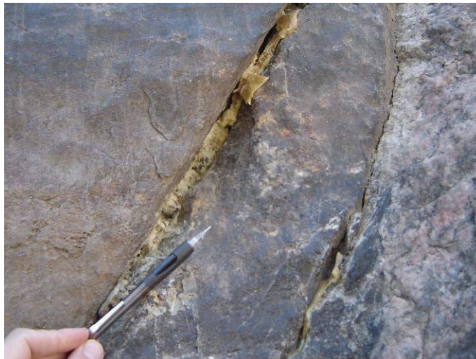
Figure 49. Photo. Polyurethane resin used in a fracture, Poudre Canyon, Colorado.
