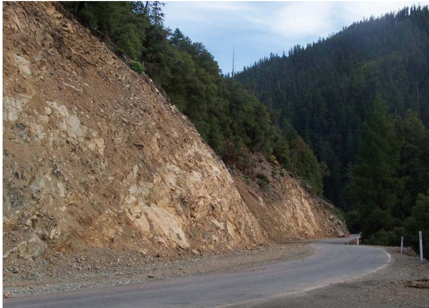
Figure 30. Photo. Drainage intercept layback cut into a slope, Hyampom Road, California.
