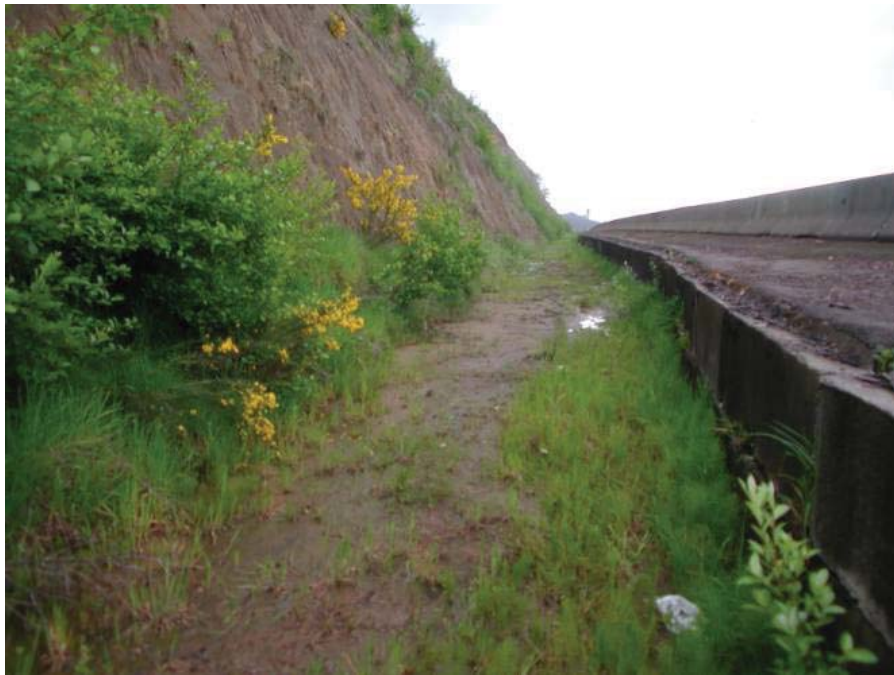
Figure 72. Photo. A hybrid ditch design.
