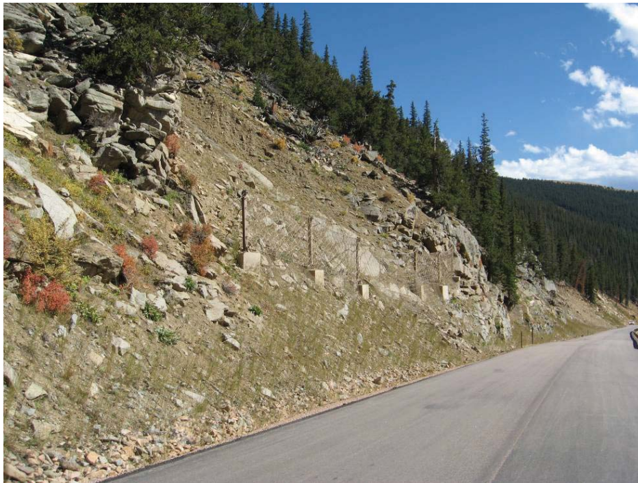
Figure 64. Photo. Installation of a flexible rockfall barrier on Guanella Pass, Colorado.
