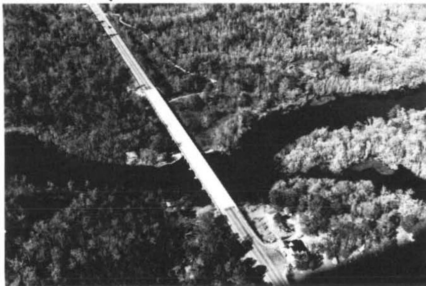
FIGURE 22 - UTILITY LINE (R.M. 49.2) (WITH U. S. 17A HIGHWAY BRIDGE) (FROM REPORT 03)
