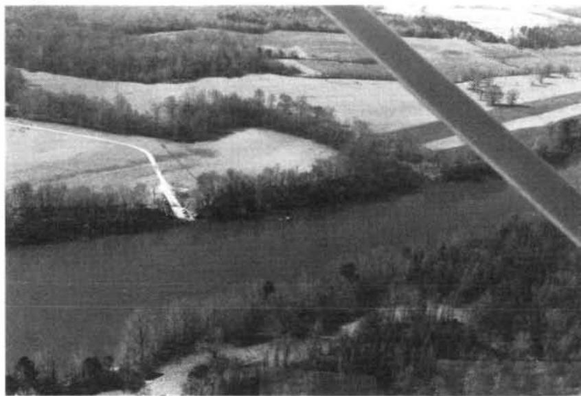
FIGURE 13 - UTILITY LINE (R.M. 68.9)
