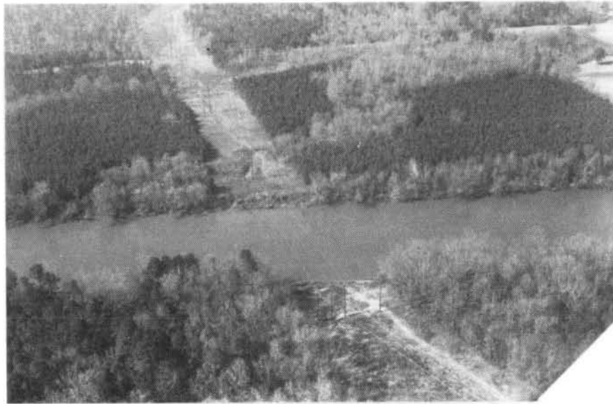
FIGURE 14 - TWO UTILITY LINES (R.M. 71.4)
