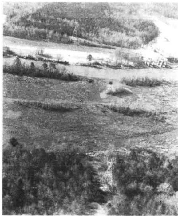
FIGURE 15 - UTILITY LINE (R.M. 75.9)
