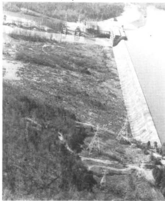
FIGURE 16 - TWO UTILITY LINES AND DAM (R.M. 76.1)
