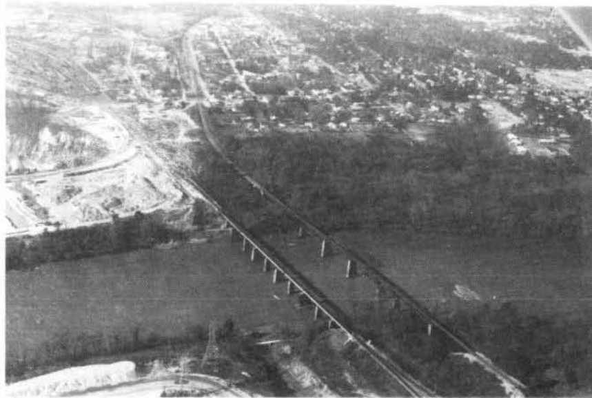
FIGURE 11 - UTILITY LINE (R.M. 174.3) (AND SEABOARD COAST LINE RAILROAD AND SOUTHERN RAILROAD BRIDGES)
