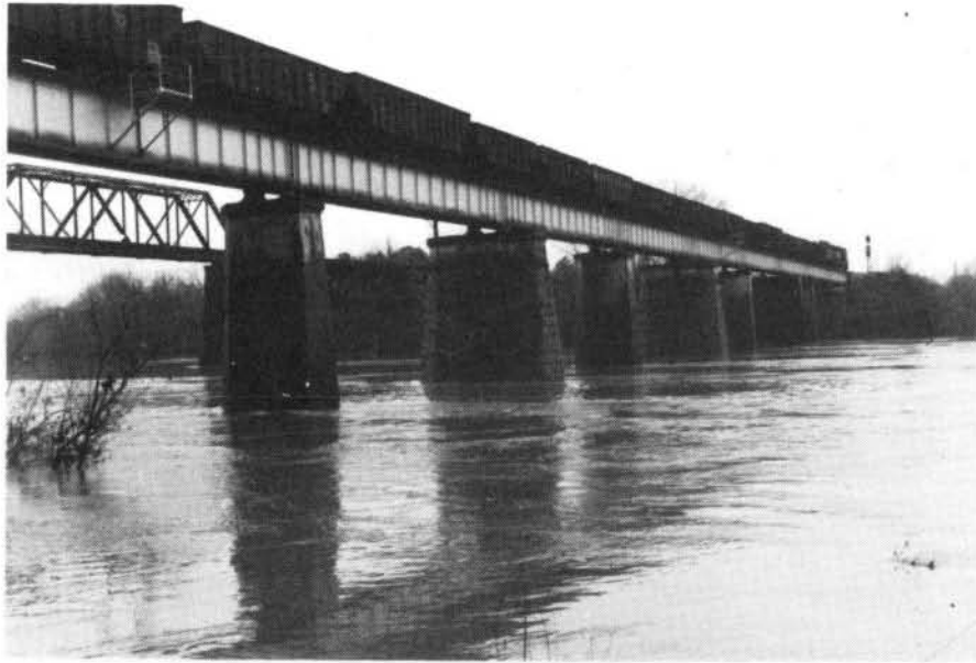
FIGURE 12 - SEABOARD COAST LINE RAILROAD BRIDGE (R.M. 174.4)
