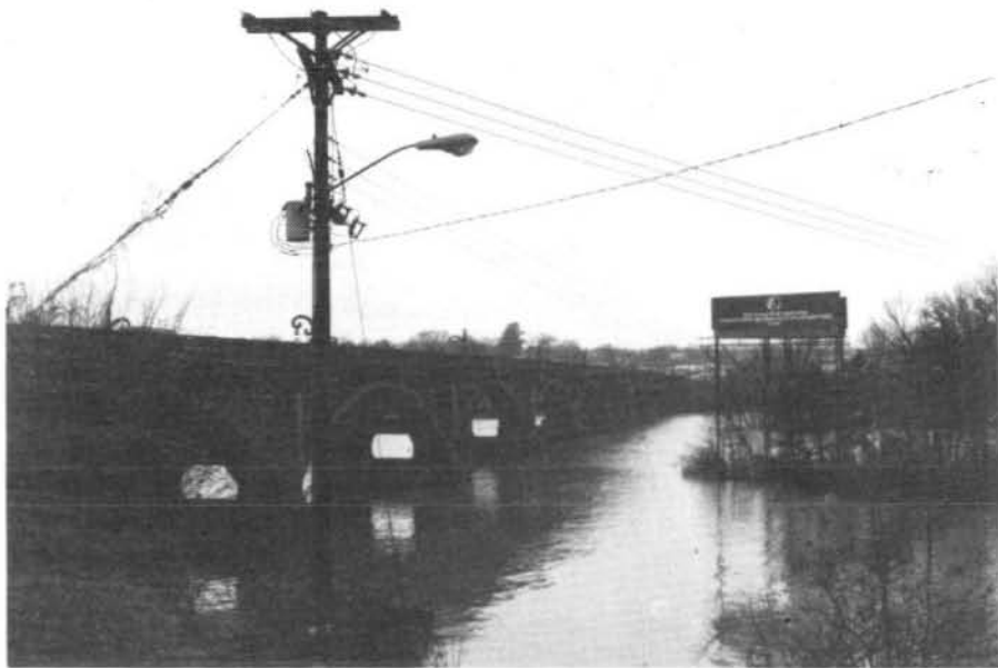
FIGURE 15 - U. S. 378-1 HIGHWAY BRIDGE (R.M. 175.9)
