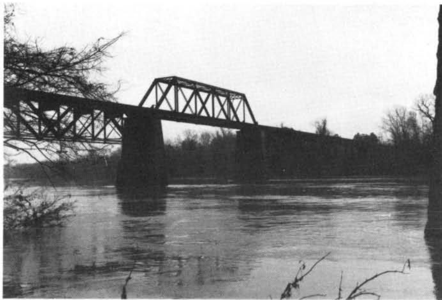
FIGURE 13 - SOUTHERN RAILROAD BRIDGE (R.M. 174.4)
