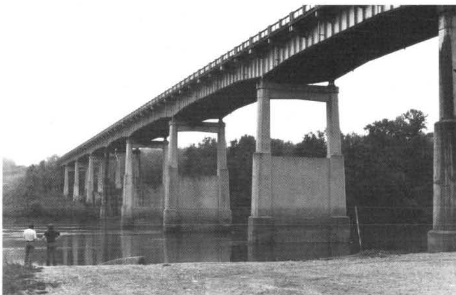
FIGURE 3 - U. S. 601 HIGHWAY BRIDGE (R.M. 127.1)
