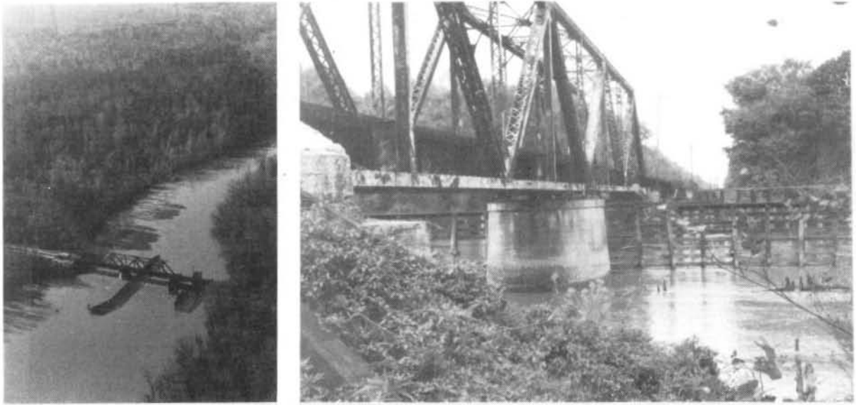
FIGURE 4 - SOUTHERN RAILROAD BRIDGE (R.M. 129.8)
