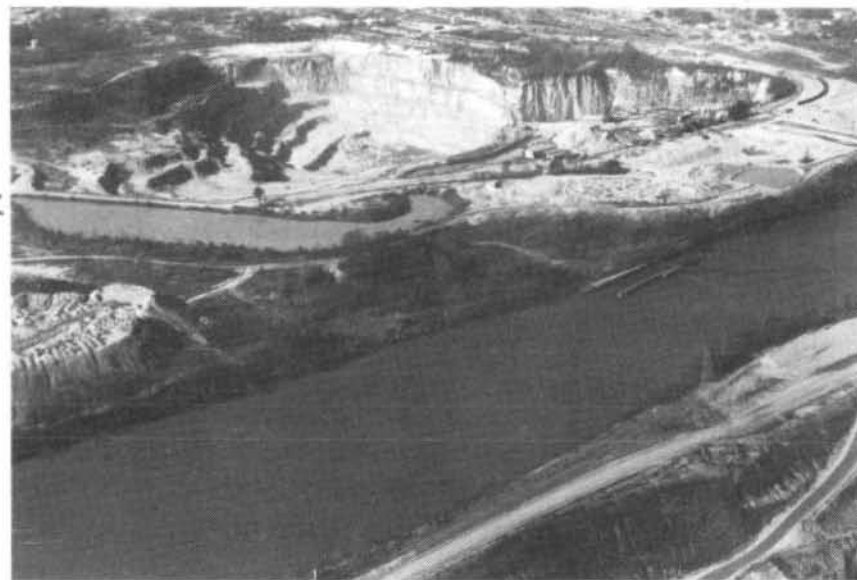
FIGURE 9 - TWO UTILITY LINES (R.M. 173.9)
