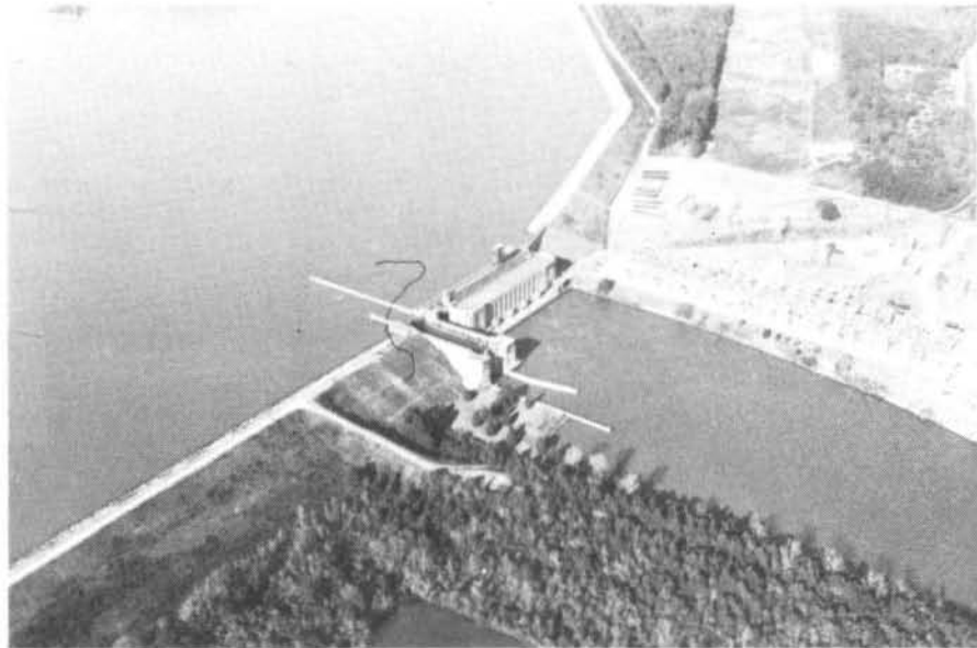
FIGURE 6 - PINOPOLIS LOCK AND DAM (R.M. 48.1)
