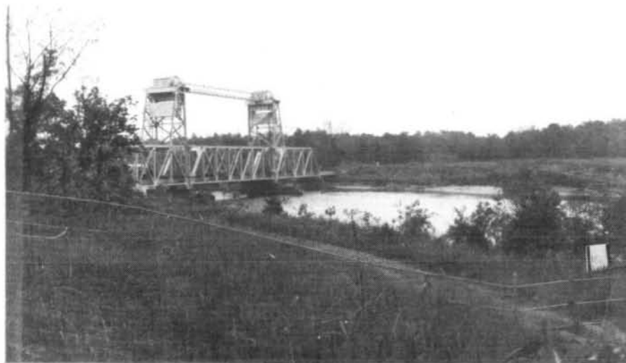
FIGURE 5 - SEABOARD COAST LINE RAILROAD BRIDGE (R.M. 47.4) (UTILITY LINE)
