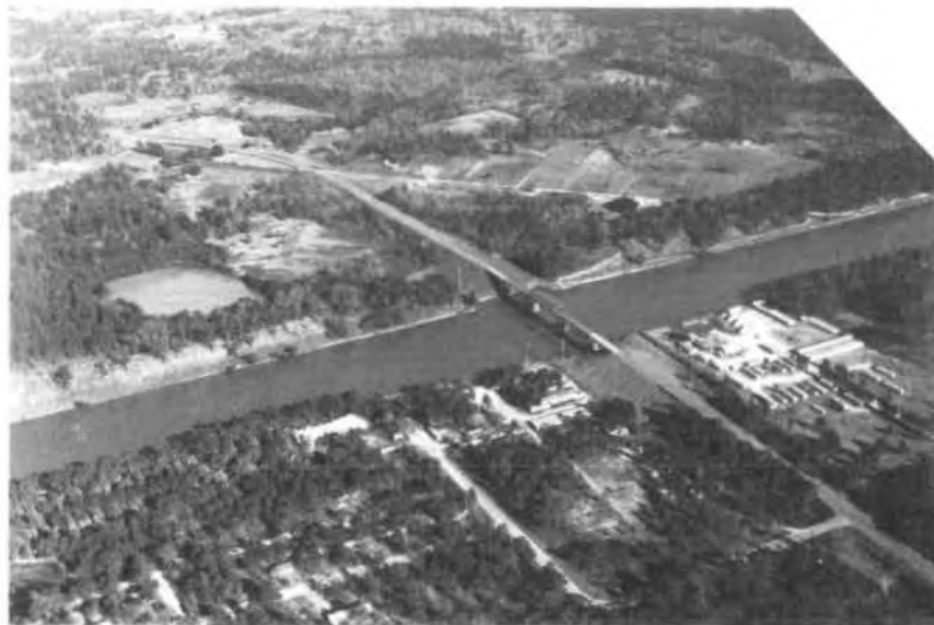
FIGURE 3 - S. C. 45 HIGHWAY BRIDGE (DIVERSION CANAL)
