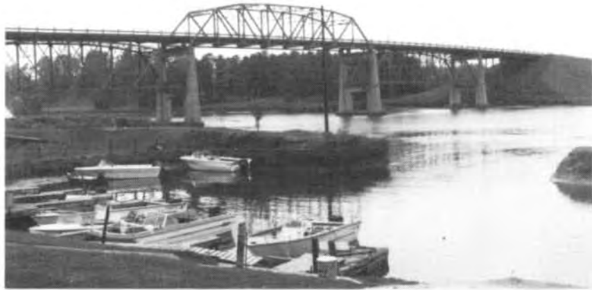
FIGURE 4 - S. C. 45 HIGHWAY BRIDGE (DIVERSION CANAL)
