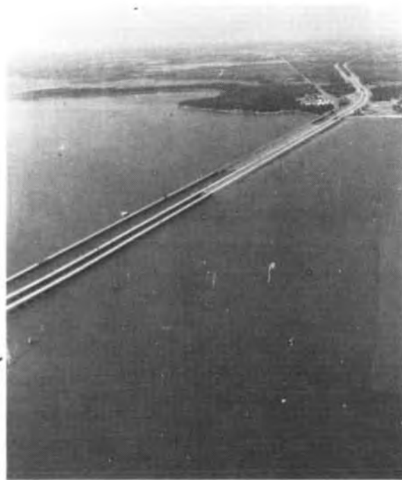
FIGURE 6 - INTERSTATE 95, U. S. 15 HIGHWAY BRIDGES (AND POWER LINE) (LAKE MARION 18-03)
