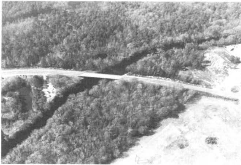
FIGURE 18 - UTILITY LINE (R.M. 62.1) (AND N. C. SECONDARY 2202 HIGHWAY BRIDGE)
