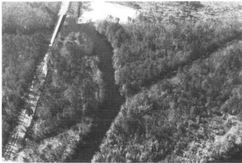
FIGURE 17 - UTILITY LINE (R.M. 60.3) (AND N. C. SECONDARY 1620 HIGHWAY BRIDGE)
