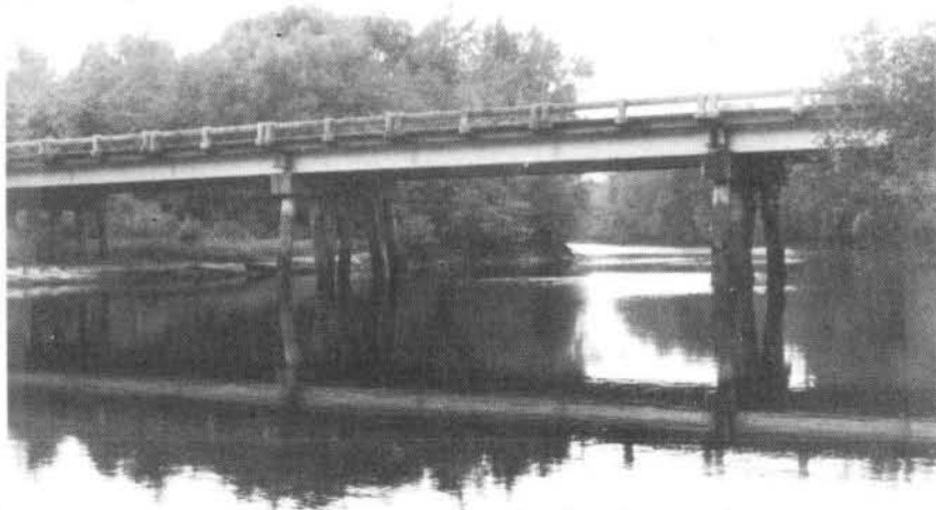
FIGURE 8 - U. S. 74, N. C. 130 HIGHWAY BRIDGE (R.M. 39.9)
