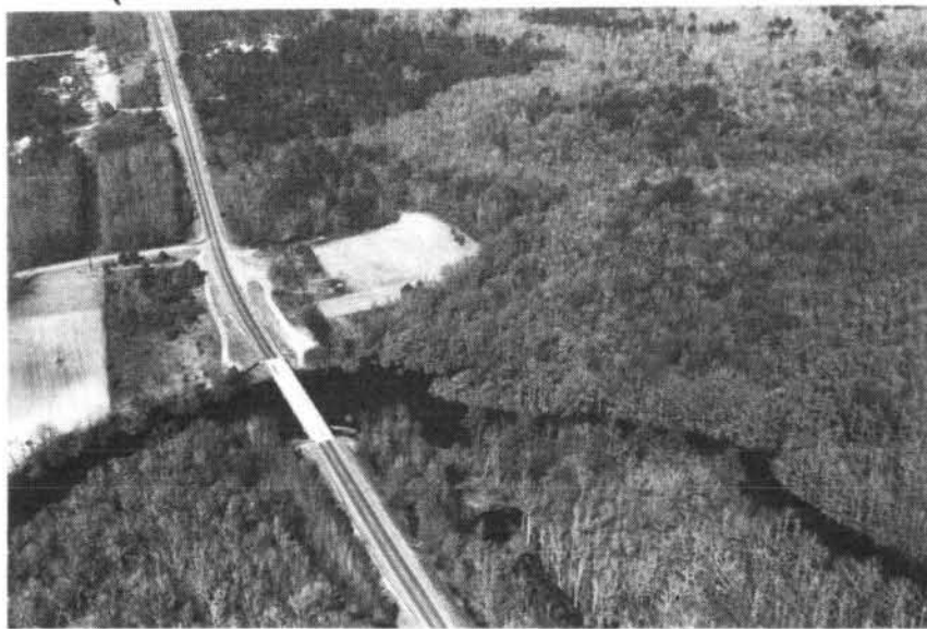
FIGURE 9 - UTILITY LINE (R.M. 40.0) (AND U. S. 74, N. C. 130 HIGHWAY BRIDGE)
