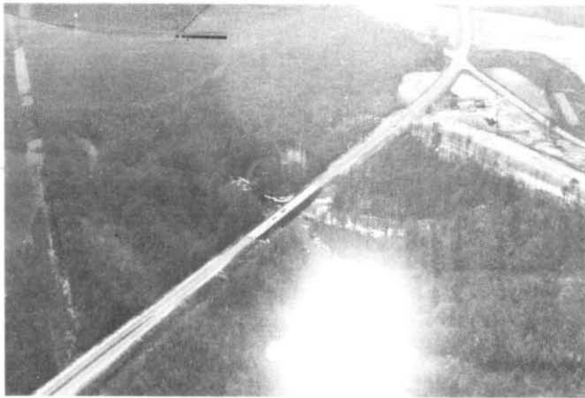
FIGURE 20 - UTILITY LINE (R.M. 62.5) (AND N. C. SECONDARY 2289 HIGHWAY BRIDGE)
