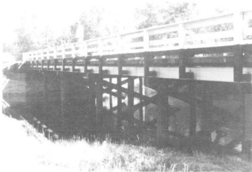
FIGURE 19 -- N. C. SECONDARY 2202 HIGHWAY BRIDGE (R.M. 62.1)
