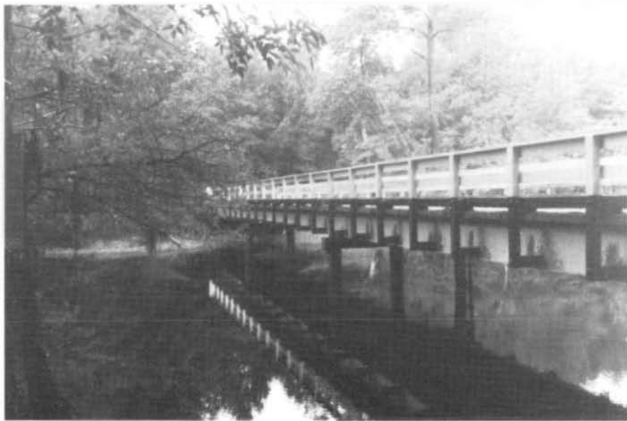
FIGURE 11 - N. C. SECONDARY 2123 HIGHWAY BRIDGE (R.M. 52.6)
