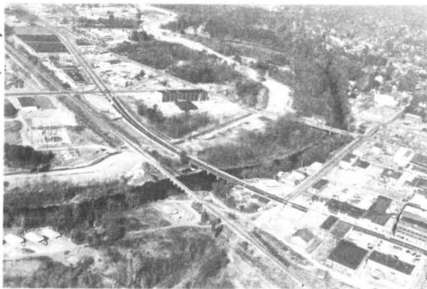
FIGURE 25 - TWO UTILITY LINES (R.M. 63.3 & 63.4) (AND SEABOARD COAST LINE RAILROAD BRIDGE & N. C. 41 HIGHWAY BRIDGE)
