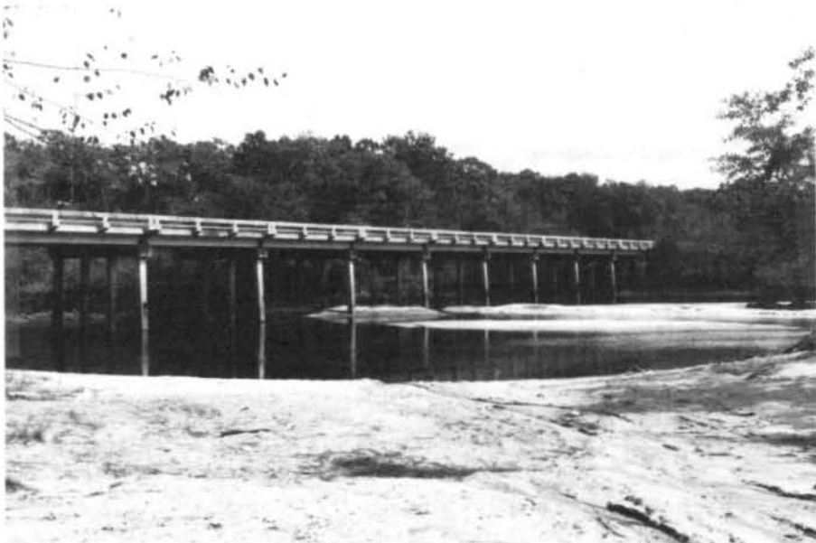
FIGURE 3 - U. S. 76, S. C. 9 HIGHWAY BRIDGE (R.M. 4.8)
