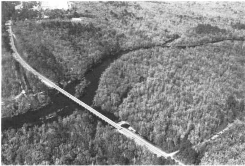
FIGURE 2 - TWO UTILITY LINES (R.M. 4.8) (AND U. S. 76, S. C. 9 HIGHWAY BRIDGE)
