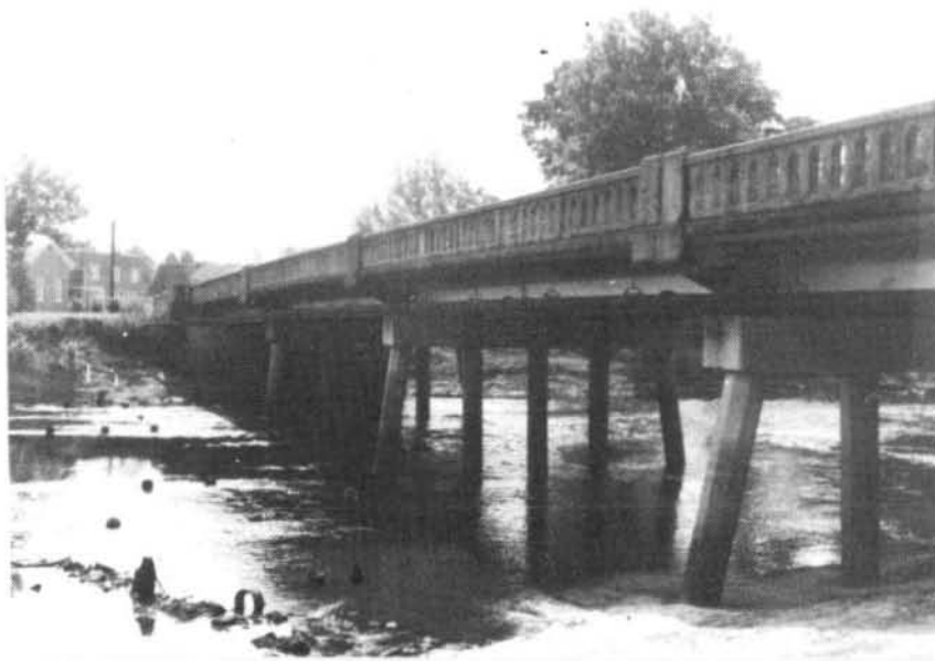
FIGURE 6 - N. C. 904 HIGHWAY BRIDGE (R.M. 20.1)
