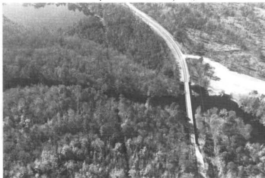
FIGURE 15 - THREE UTILITY LINES (R.M. 60.1, 60.2, & 60.2) (AND N. C. SECONDARY 1620 HIGHWAY BRIDGE)
