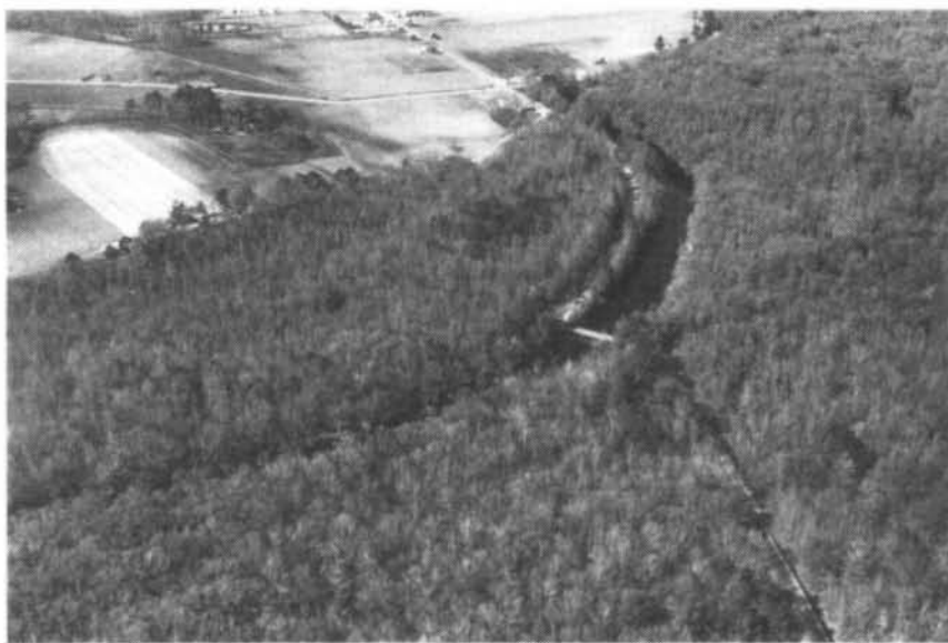
FIGURE 12 - N. C. SECONDARY 2123 HIGHWAY BRIDGE (R.M. 52.6)
