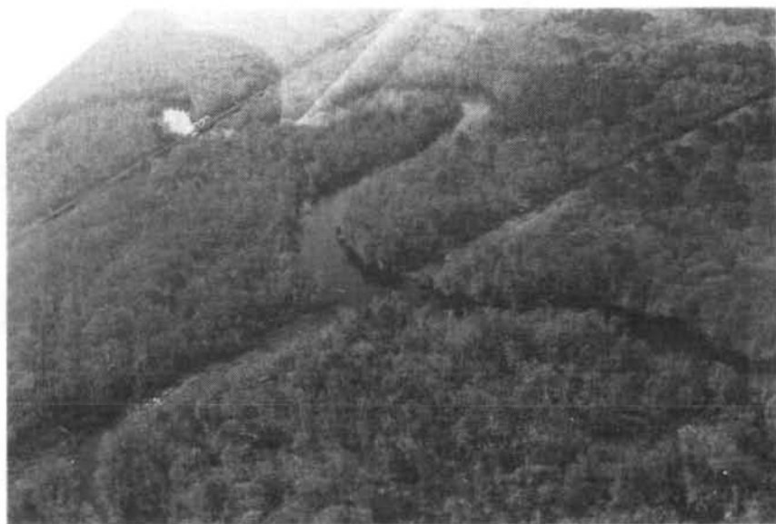
FIGURE 5 - UTILITY LINE (R.M. 7.4)
