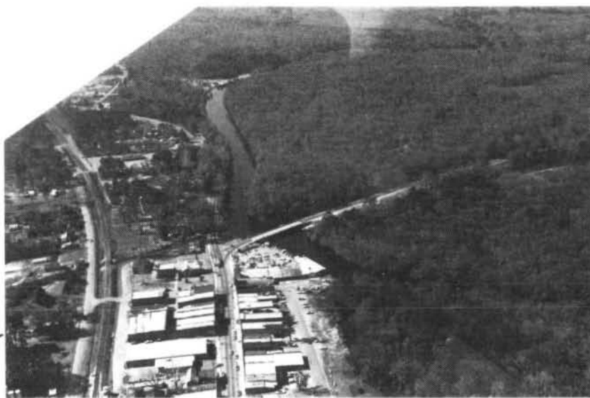
FIGURE 7 - UTILITY LINE (R.M. 20.1) (AND N. C. 904 HIGHWAY BRIDGE)
