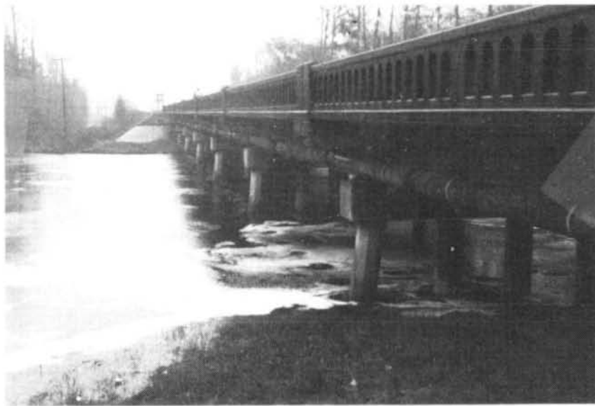
FIGURE 22 - N. C. SECONDARY 2289 HIGHWAY BRIDGE (R.M. 62.6)
