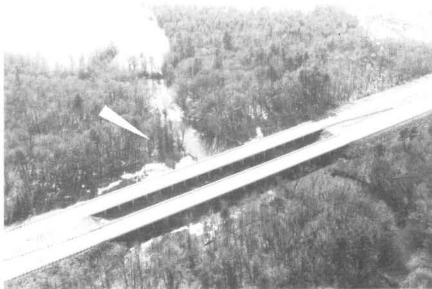
FIGURE 31 - INTERSTATE 20 HIGHWAY BRIDGES (R.M. 92.9)
