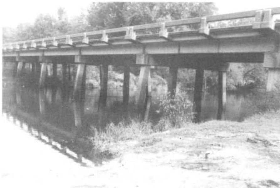
FIGURE 28 - U. S. 401 HIGHWAY BRIDGE (R.M. 84.6)
