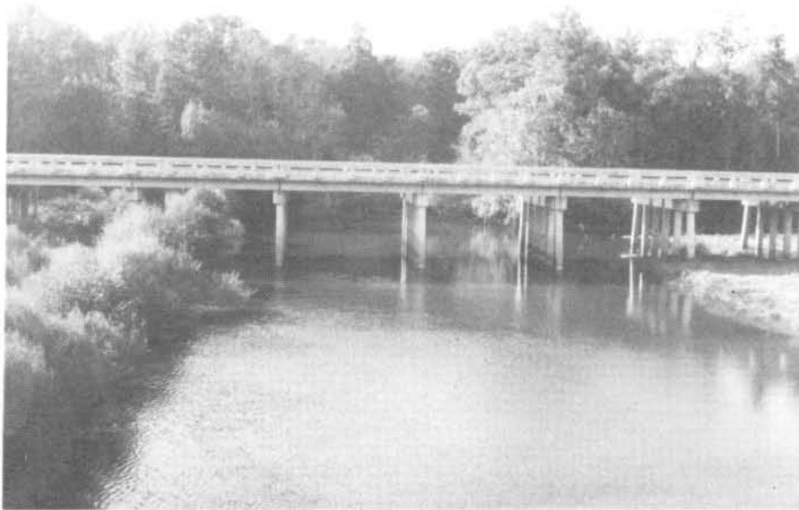
FIGURE 22 - INTERSTATE 95 HIGHWAY BRIDGE (NORTH BOUND) (R.M. 67.5)
