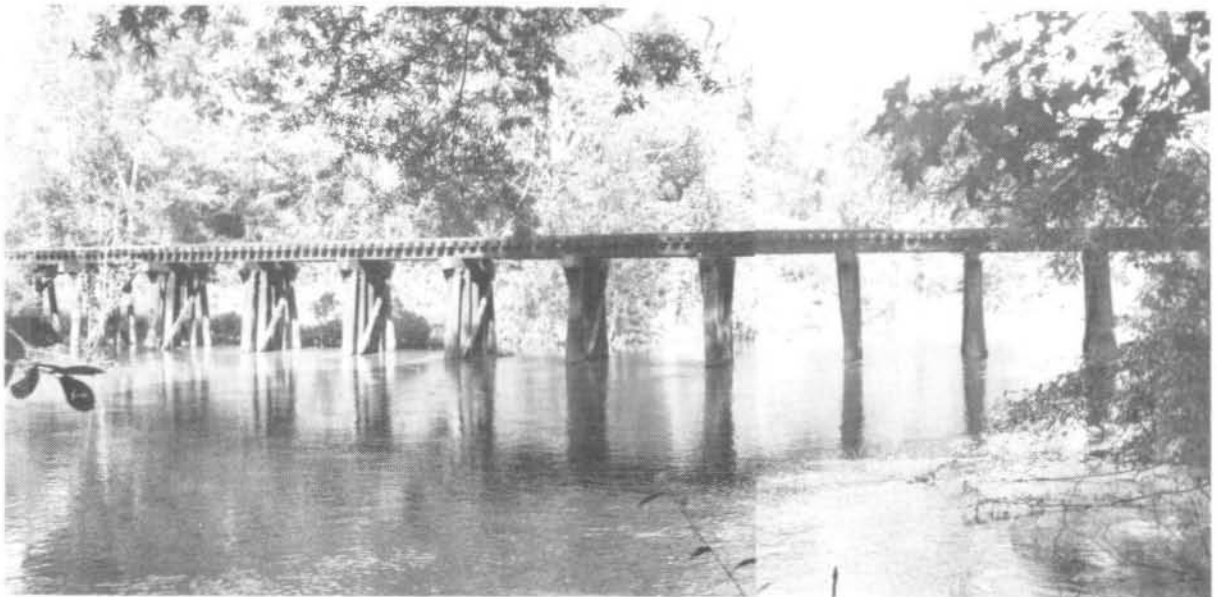
FIGURE 35 - SEABOARD COAST LINE RAILROAD BRIDGE (R.M. 98.3)
