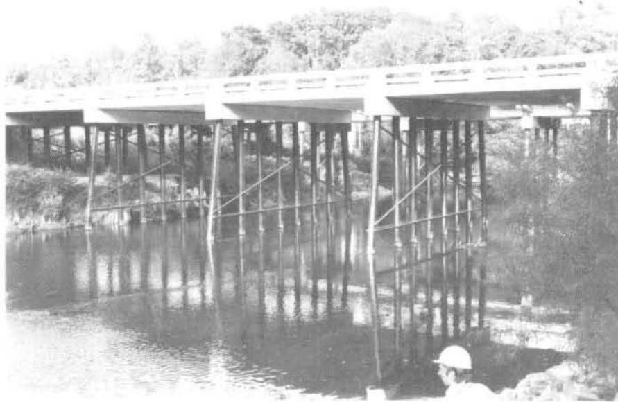
FIGURE 14 - U. S. 52 HIGHWAY BRIDGE (SOUTH BOUND) (R.M. 42.5)
