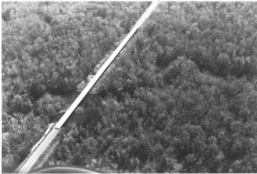
FIGURE 20 - UTILITY LINE (R.M. 64.4) (AND U. S. 403 HIGHWAY BRIDGE)
