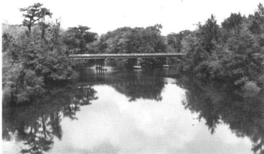
FIGURE 4 - S. C. 41 AND S. C. 51 HIGHWAY BRIDGE (R.M. 6.5)
