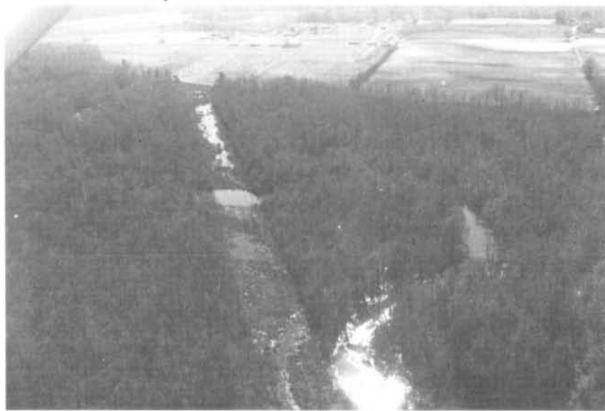
FIGURE 18 - UTILITY LINE (R.M. 59.3)
