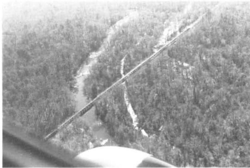
FIGURE 34 - SEABOARD COAST LINE RAILROAD BRIDGE (R.M. 98.3)
