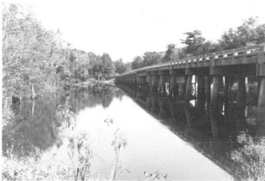
FIGURE 7 - S. C. SECONDARY 49 HIGHWAY BRIDGE (R.M. 15.4)
