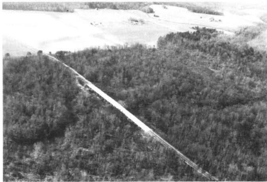
FIGURE 38 - S. C. SECONDARY 17 HIGHWAY BRIDGE (R.M. 108.3)
