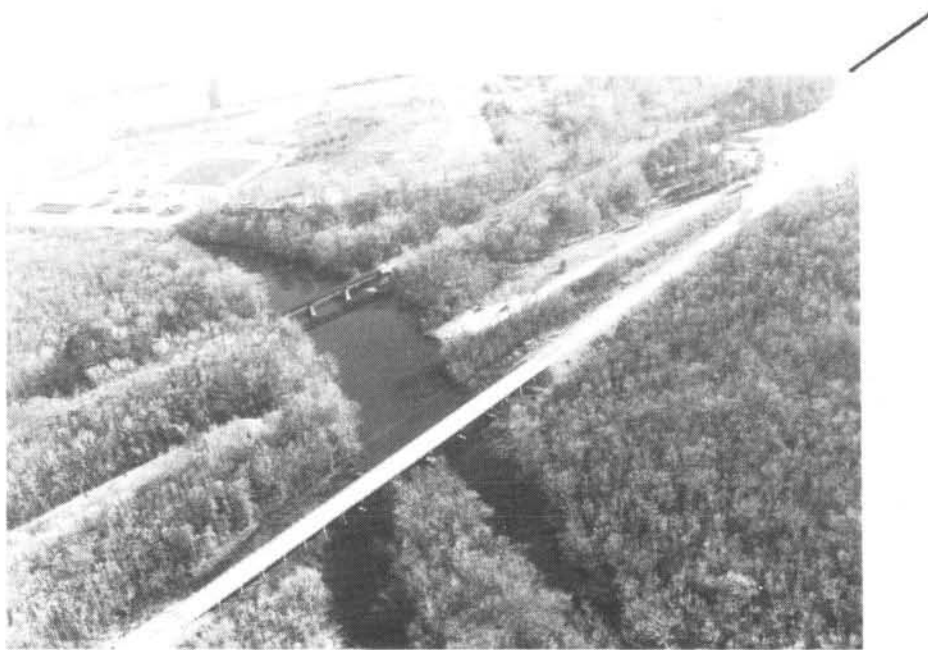
FIGURE 3 - UTILITY LINE (R.M. 6.5) (AND SCLRR BRIDGE AND S. C. 41 AND 51 HIGHWAY BRIDGE)
