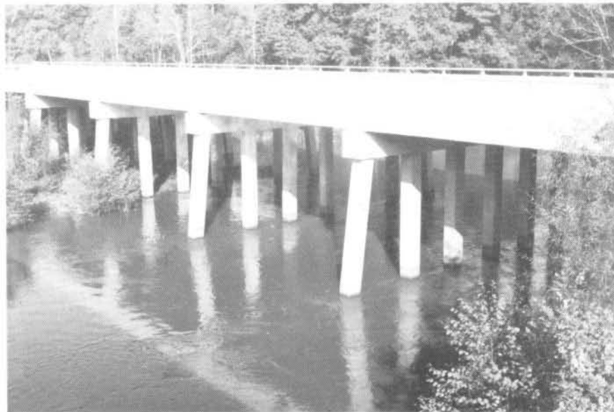
FIGURE 33 - INTERSTATE 20 HIGHWAY BRIDGE (WEST BOUND) (R.M. 92.9)
