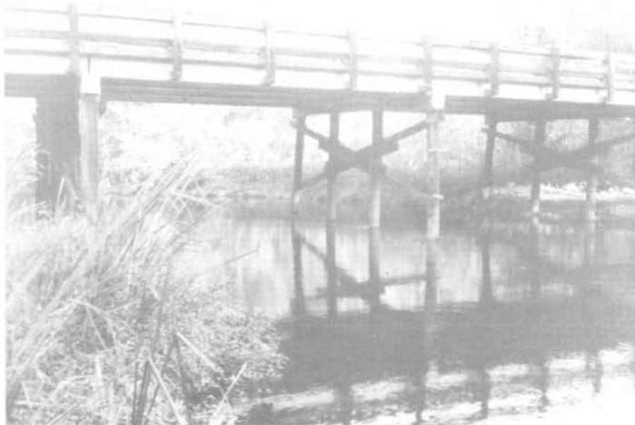
FIGURE 19 - U. S. 403 HIGHWAY BRIDGE (R.M. 64.4)
