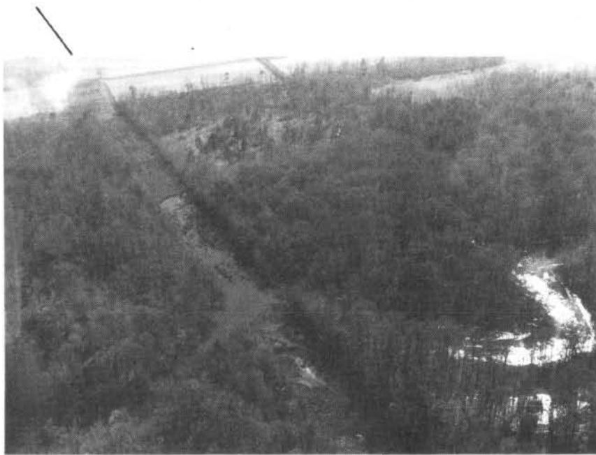
FIGURE 16 - UTILITY LINE (R.M. 53.9)
