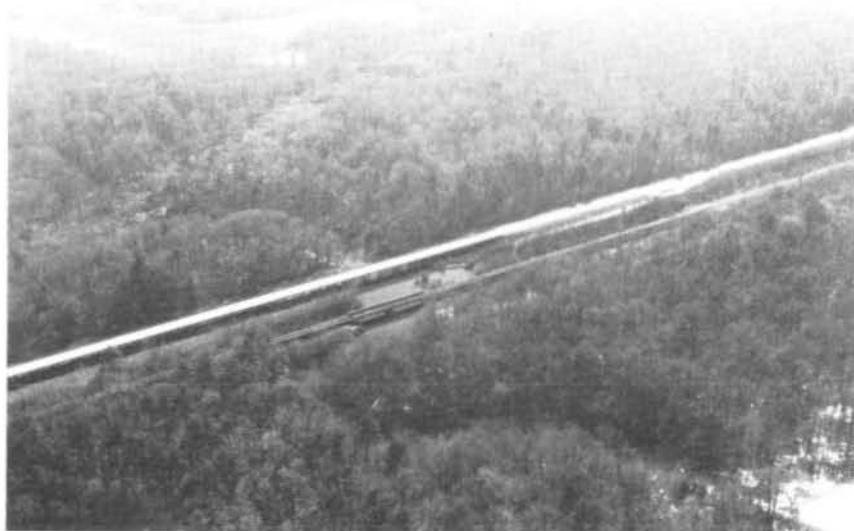
FIGURE 25 - U. S. 76 HIGHWAY BRIDGE AND SCLRR BRIDGE (R.M. 74.5)
