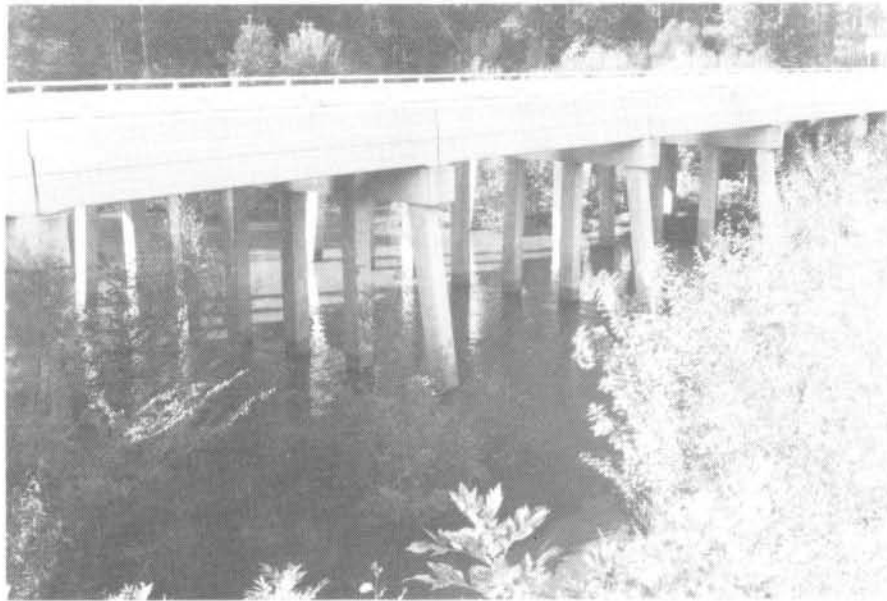
FIGURE 32 - INTERSTATE 20 HIGHWAY BRIDGE (EAST BOUND) (R.M. 92.9)
