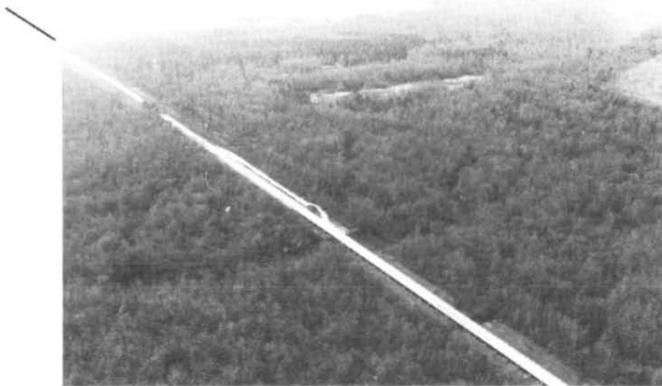
FIGURE 29 - UTILITY LINE (R.M. 84.6) (AND U. S. 401 HIGHWAY BRIDGE)
