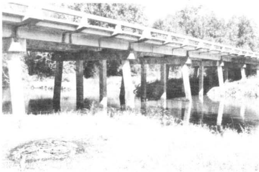
FIGURE 41 - S. C. SECONDARY 15 AND S. C. SECONDARY 23 HIGHWAY BRIDGE (R.M. 114.3)
