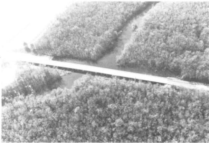
FIGURE 6 - UTILITY LINE (R.M. 15.4) (AND S. C. SECONDARY 49 HIGHWAY BRIDGE)
