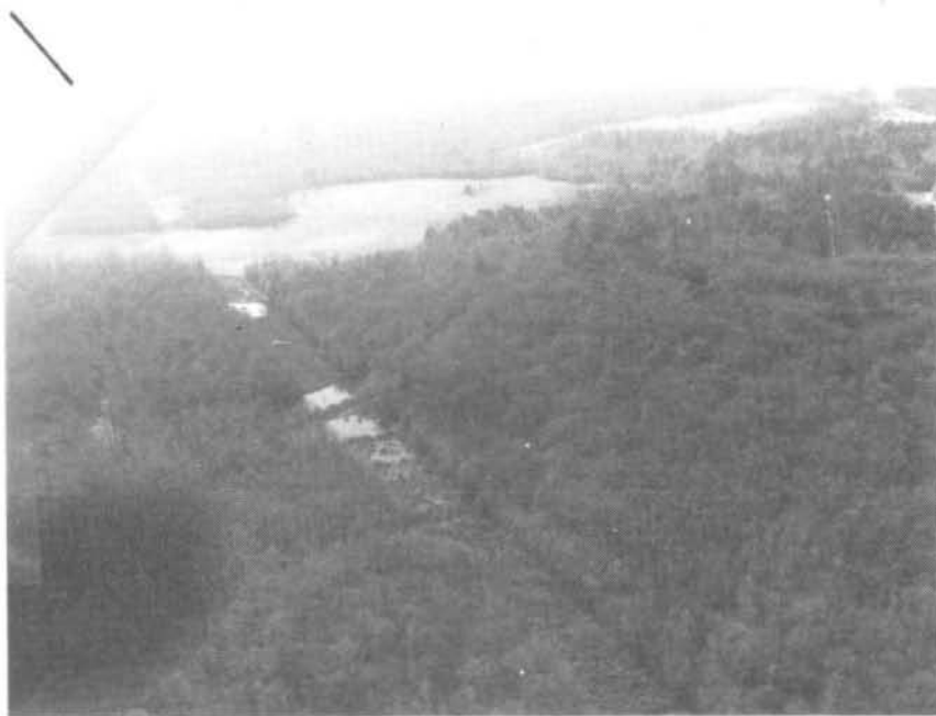
FIGURE 10 - UTILITY LINE (R.M. 30.6)
