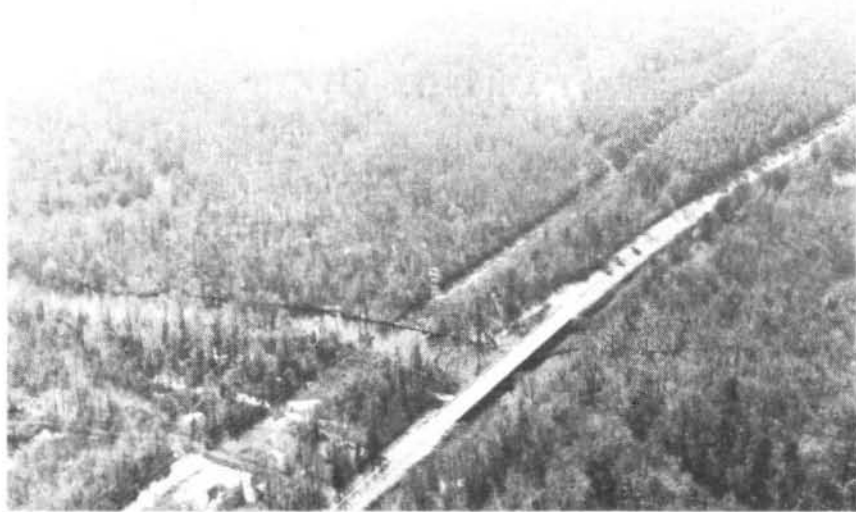
FIGURE 40 - UTILITY LINE (R.M. 114.3) (AND S. C. SECONDARY 15 AND S. C. SECONDARY 23 HIGHWAY BRIDGE)
