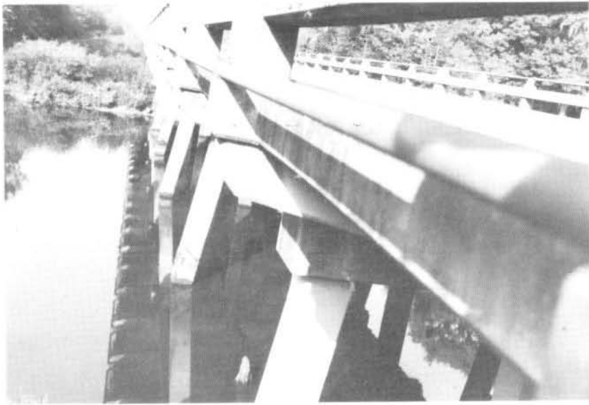
FIGURE 8 - U. S. 378 HIGHWAY BRIDGE (R.M. 27.6)
