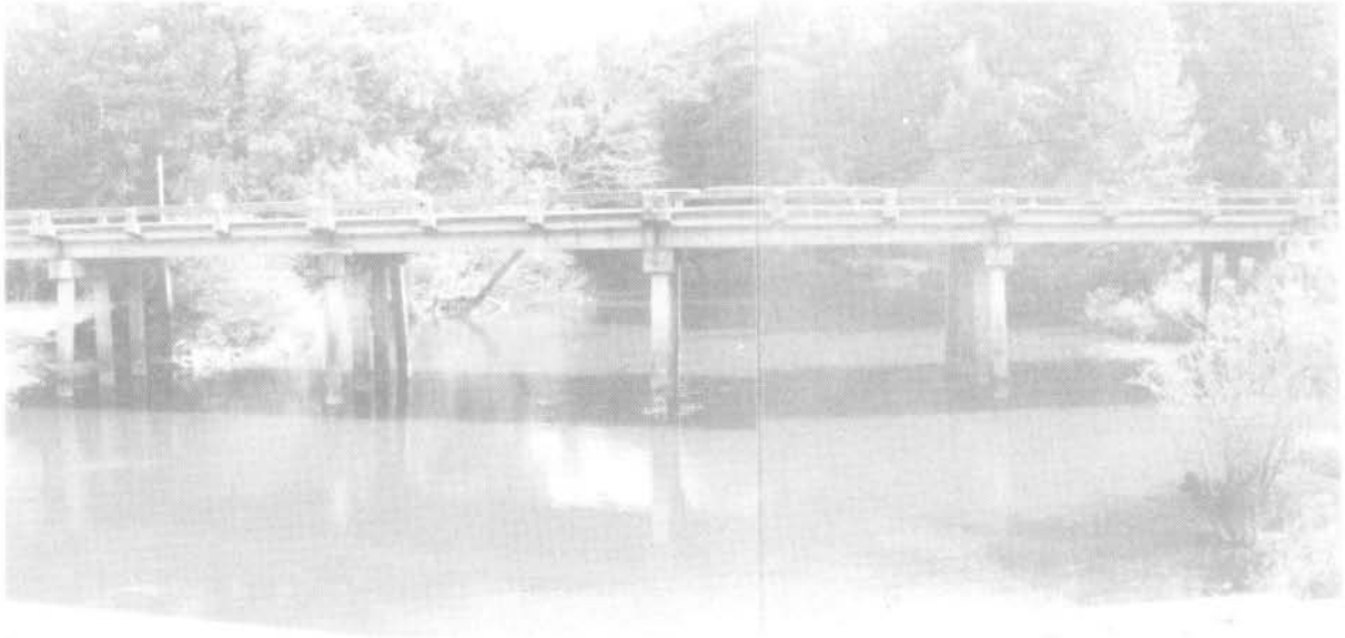
FIGURE 26 - U. S. 76 HIGHWAY BRIDGE (R.M. 74.5)
