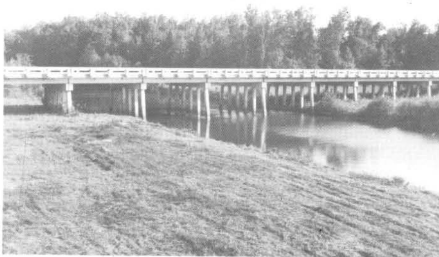
FIGURE 23 - INTERSTATE 95 HIGHWAY BRIDGE (SOUTH BOUND) (R.M. 67.5)
