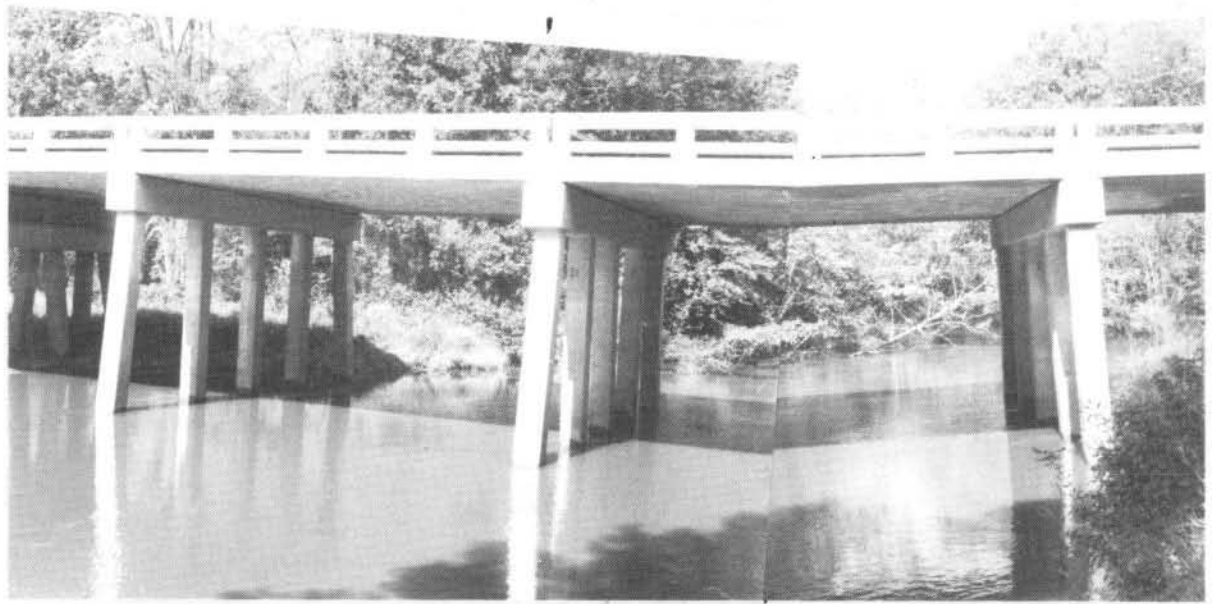
FIGURE 39 - S. C. SECONDARY 17 HIGHWAY BRIDGE (R.M. 108.3)
