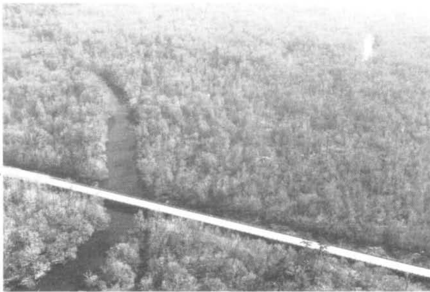
FIGURE 9 - UTILITY LINE (R.M. 27.6) (AND U. S. 378 HIGHWAY BRIDGE)
