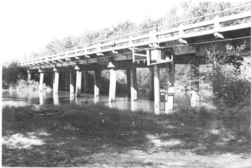
FIGURE 37 - U. S. 15 AND S. C. 34 HIGHWAY BRIDGE (R.M. 99.4)
