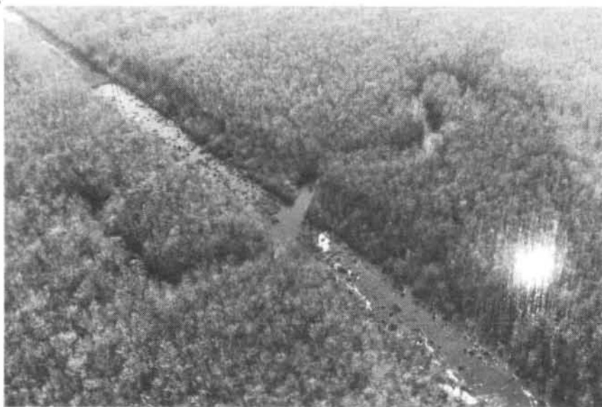
FIGURE 5 - UTILITY LINE (R.M. 8.0)
