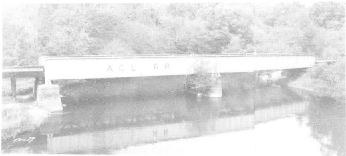
FIGURE 27 - SEABOARD COAST LINE RAILROAD BRIDGE (R.M. 74.5)
