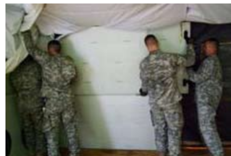
Soldiers installing Modular Ballistic Protective System (MBPS), a lightweight armor system installed directly into existing military shelters where Warfighters work, eat and live
