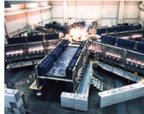
Shiva Star - AFRL's High-Power Systems Facility on Kirtland AFB, New Mexico.
