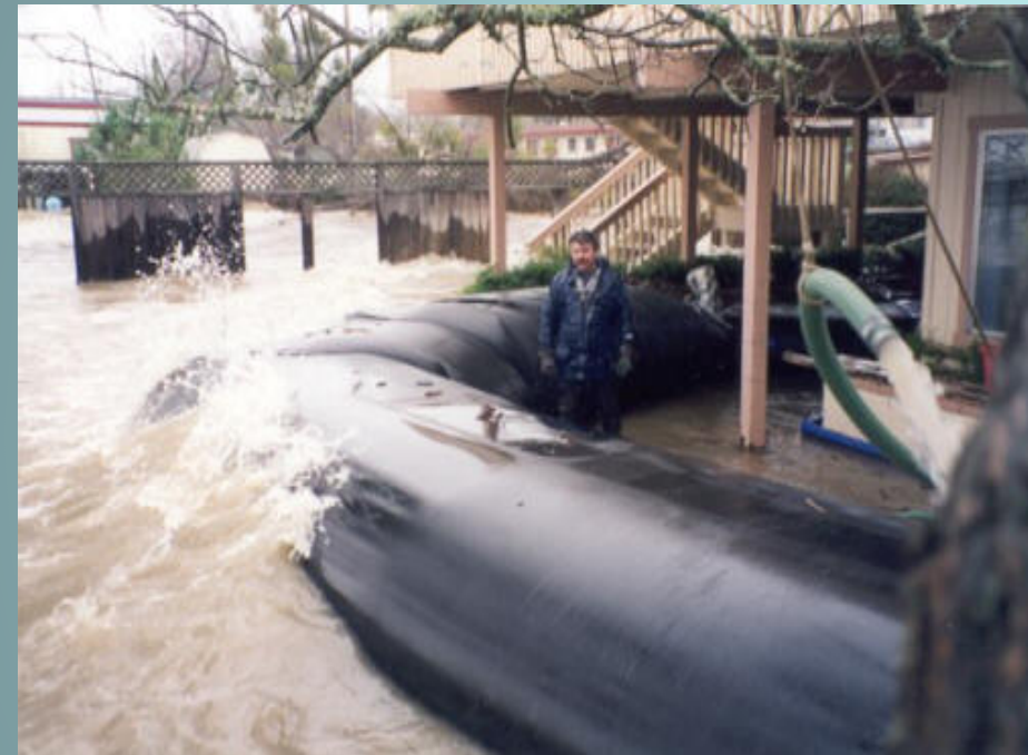
Water-filled cofferdams
