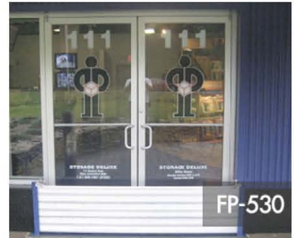
Example of Manually-Installed Panel
