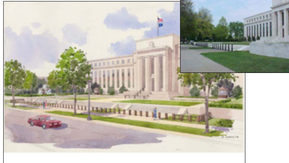
The Eccles Building along Constitution Avenue, NW
