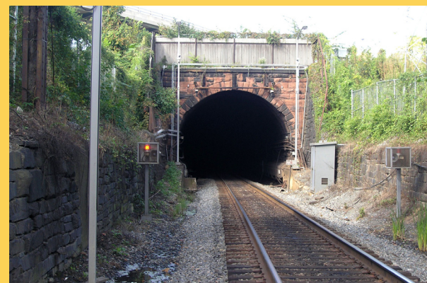
Figure 2-5. Virginia Avenue Tunnel
