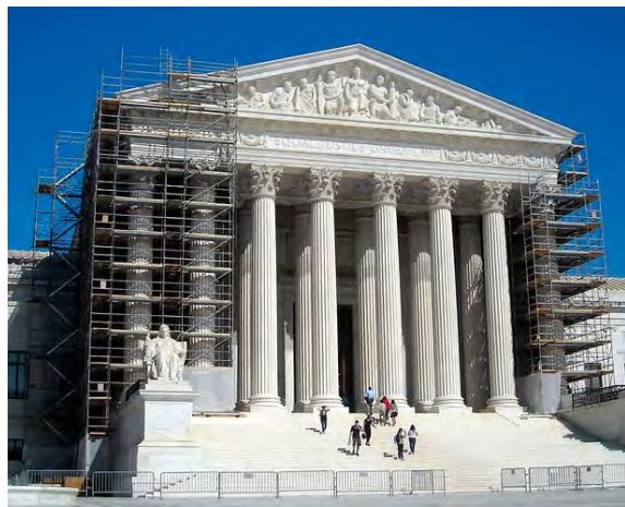
Restoration of the Supreme Court Building.
