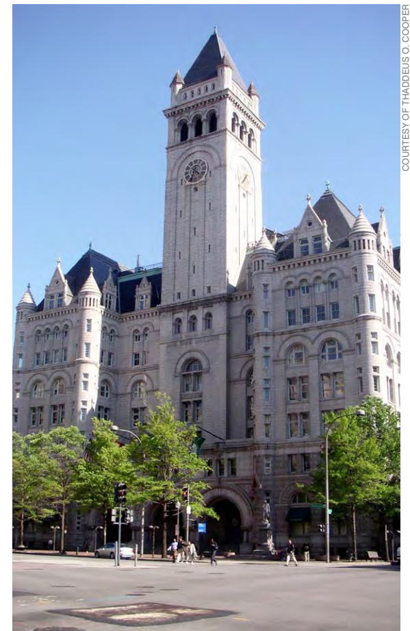
Current view of the Old Post Office Building located on Pennsylvania Avenue between the White House and U.S. Capitol.
