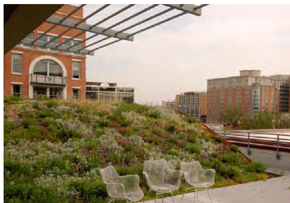
Green roofs will minimize stormwater runoff, help reduce the heat island effect, and provide urban amenities.
