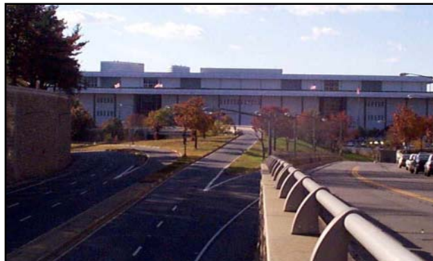
The image above looks west from E Street to the Kennedy Center. Proposals to reconfigure the E Street Expressway interchange could include an area for the development of an urban plaza that could incorporate a memorial and/or flanking museums.
