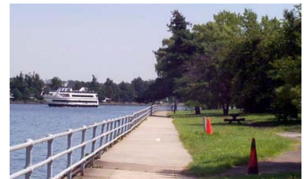
Washington Channel shoreline provides an appropriate landscape setting for a future commemorative feature that would reflect the parkland context of East Potomac Park's waterfront.
