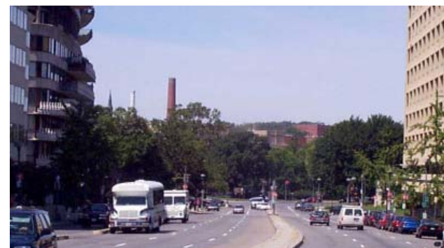
Waterfront setting on the Potomac River and Rock Creek shown in the distance provides opportunities for a future prominent commemorative feature that could be located on axis with Virginia Avenue.
