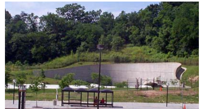
One potential site associated with the Fort Totten Metro station is located above the tunnel retaining wall on a prominent slope with a wooded setting.
