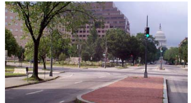
Direct views of Capitol from these triangular park areas are possible along New Jersey Avenue. The parks offer prominent settings for appropriately scaled memorial features.
