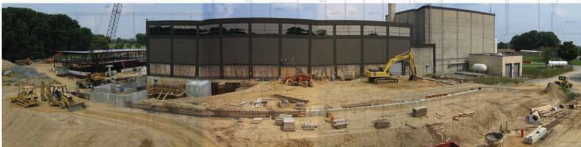
Panoramic view of New Guide Hall construction
