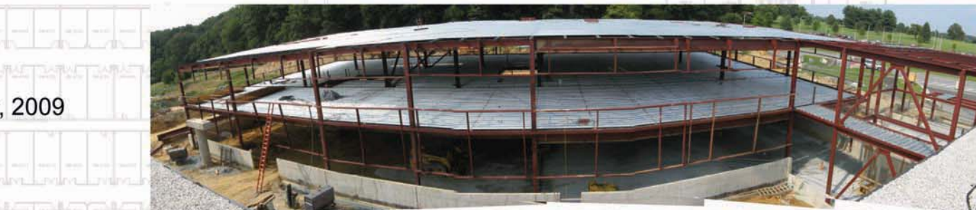
Panoramic view of Technical Support Building construction
