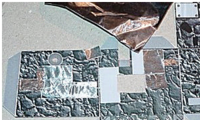
Aluminium foil fitted as coolers on the panels
