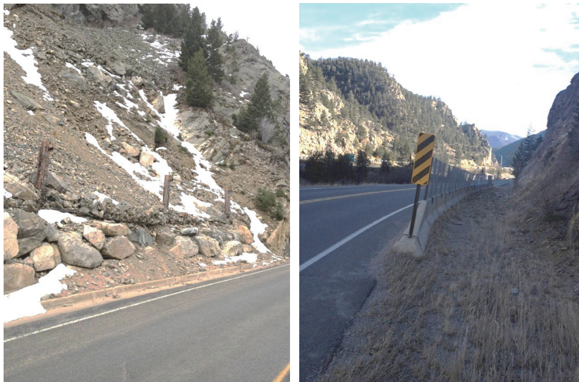
Figure 6. Photos. Example rockfall fence installations.
