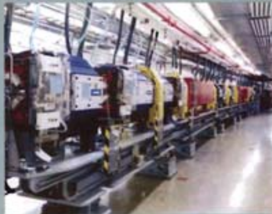
Image 15. Advanced Photon Source (APS) storage ring sector. (Photo Courtesy of Argonne National Laboratory.)
