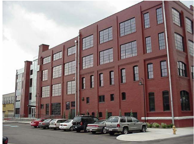
Picture of the exterior of the Wheeling Stamping Building after renovation.
