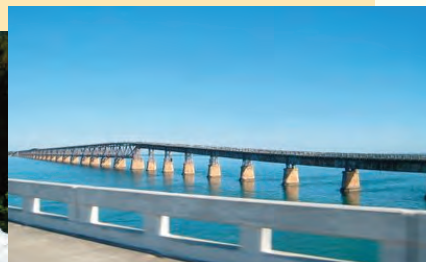
Remote network monitoring of structural health of bridges (Wikimedia Commons Jsmjr/John)
