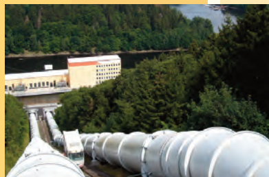
Digital imaging of pipeline damage (Wikimedia Commons/Mazbln)
