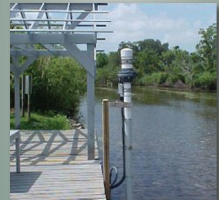
St. Charles, LA tide gauge, one component of the St. Charles Parish Water Level Monitoring System. This system will provide critical information to save lives, protect property, and restore the environment in this community. Credit: NOAA
