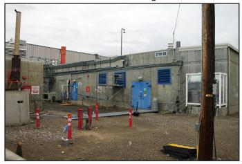
The vault complex was part of Hanford's Plutonium Finishing Plant, which produced nearly two-thirds of the nation's supply of plutonium used in the nuclear weapons program during the Cold War. Built in 1971, the vault complex held the top-secret stores of plutonium in metal canisters until they were shipped for weapons production.
