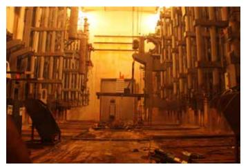
One of the buildings at the plant, called the Plutonium Reclamation Facility, includes a canyon area that houses skinny, pencil-shaped tanks mounted to racks on the walls along with other support equipment. The pencil tanks range in size from 3 feet to 22 feet long, are contaminated with plutonium and must be removed to prepare the facility for demolition. CH2M HILL will remove a total of 196 pencil tank units (racks and process equipment included).
