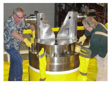
The container was then transferred to the Cold Vacuum Drying Facility adjacent to the K West Reactor where it was purged with helium gas to vacuum dry the fuel. The container was then shipped for interim storage at the Canister Storage Building until a disposal alternative is available.
