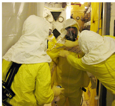
Workers prepare a glovebox inside the 242-Z facility for removal (left). Contamination inside the facility require that workers suit up in several layers of personal protective equipment (right).
