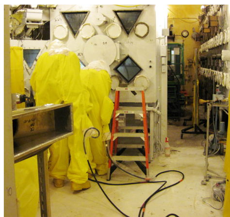
Workers prepare a glovebox inside the 242-Z facility for removal (left). Contamination inside the facility require that workers suit up in several layers of personal protective equipment (right).
