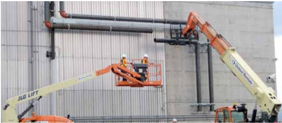
Workers install new piping and other equipment on the exterior of the 234-5Z facility (above left and right). They began construction of a new chiller system at the Plutonium Finishing Plant Complex in April. The work included installing cooling coils (middle left) and extensive internal piping (middle right) inside the facility to accommodate three new 300-ton chillers (shown staged on trailers, below) that will be installed at the facility's northeast corner.
