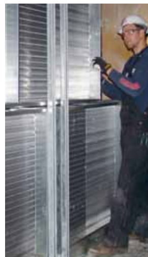
Workers install new piping and other equipment on the exterior of the 234-5Z facility (above left and right). They began construction of a new chiller system at the Plutonium Finishing Plant Complex in April. The work included installing cooling coils (middle left) and extensive internal piping (middle right) inside the facility to accommodate three new 300-ton chillers (shown staged on trailers, below) that will be installed at the facility's northeast corner.
