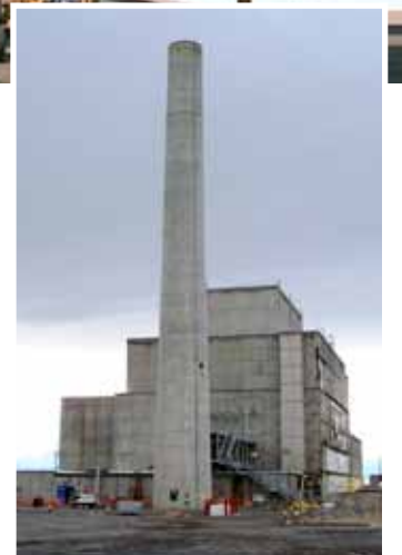
The 116-KE stack was once used to discharge ventilation gases from the K East reactor, which ceased operations in 1971. The stack was shortened from 300 feet to 175 feet in 1980-81.
