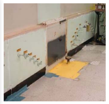
Room 153 from the Analytical Laboratories after glovebox removal.
