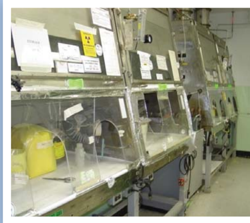
Room 153 of the Analytical Laboratories before glovebox removal.
