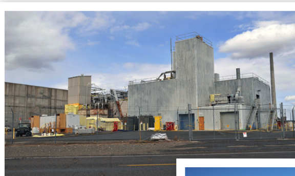
The site of the 203-UX, 224-U and 224-UA buildings before demolition
