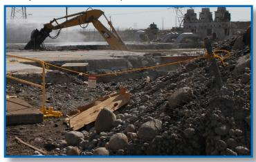
The Main Pump House, a metal-frame building that housed massive pumps and provided access to the underground pipe galleries that fed the reactor, was weakened and lowered in a matter of days. Loadout of debris from the 25,000 square foot building's remains is ongoing.
