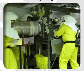
At the Plutonium Finishing Plant Remote Mechanical C Line, equipment removal and isolations are in progress on two conveyor gloveboxes that extend approximately 75 feet each through five rooms. The equipment includes waste from the "chainveyor" (a conveyor and chain mixed) that ran the length of gloveboxes HC-1 and HC-2. These are just two of 44 gloveboxes remaining gloveboxes CH2M HILL plans to remove with Recovery Act funds.
