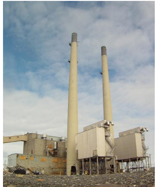
284W Power House on the Hanford Site
