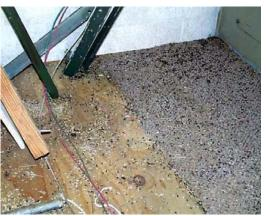
Figure 4. Heavy Rodent Contamination
