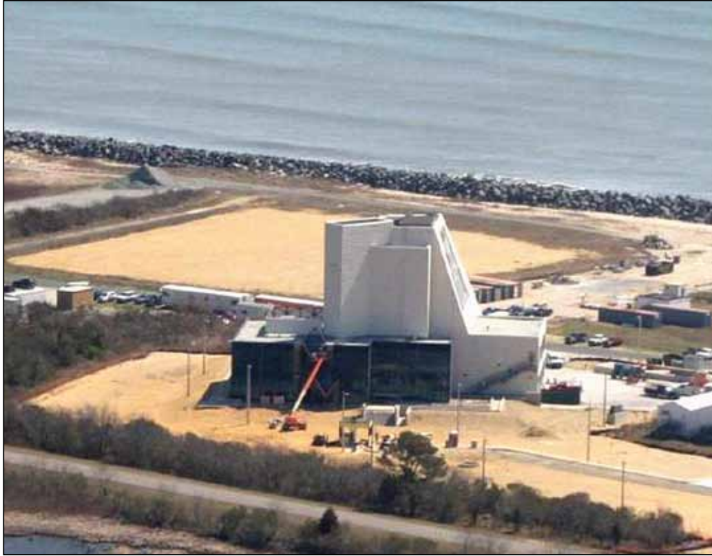
Figure 6. Dual-Band Radar Wallops Island Engineering Test Center Installation
