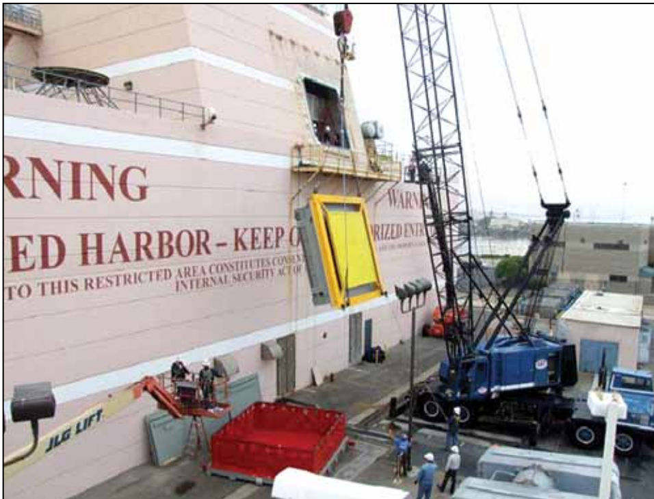
Figure 7. VSR Being Installed at the SWEF
