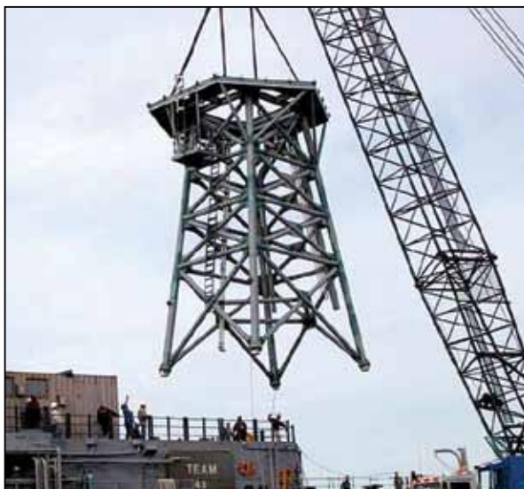
Figure 2. MFR Tower Being Installed on SDTS
