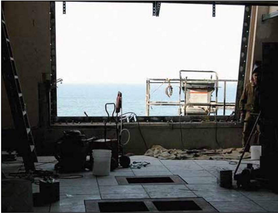
Figure 6. The Original Octagonal SPY-IA Opening Was Made Rectangular to Accommodate the VSR
