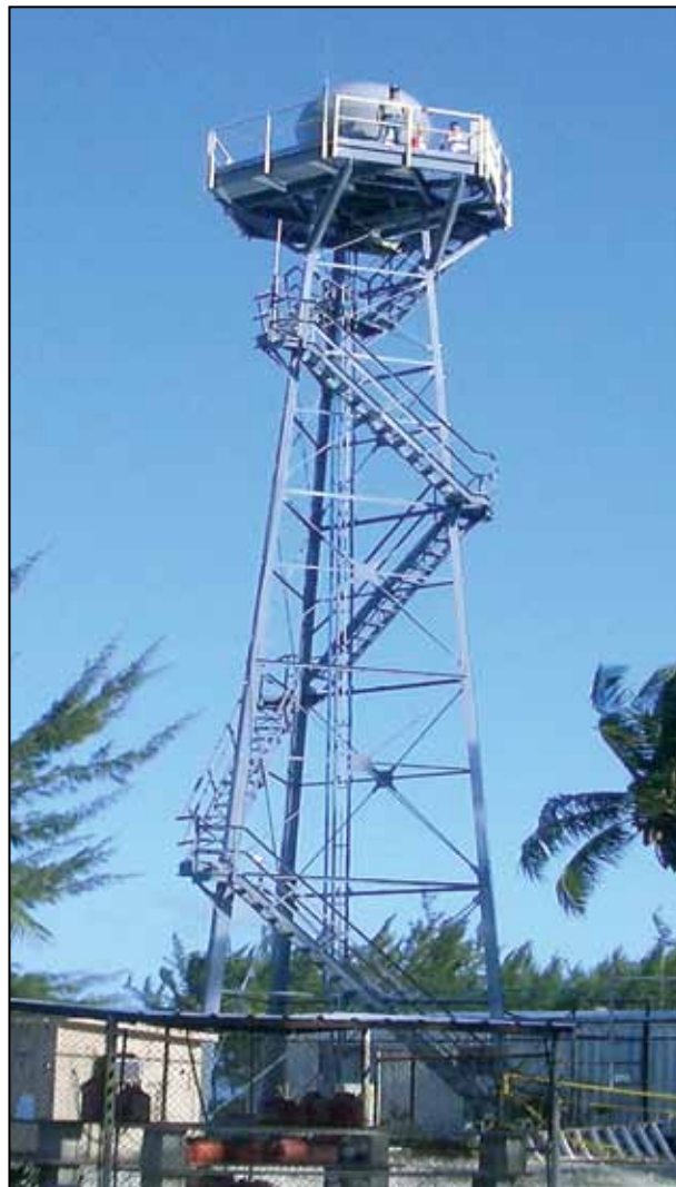
Figure 4. AN/SPS-74 Radar Installation at the AUTEC Test Site
