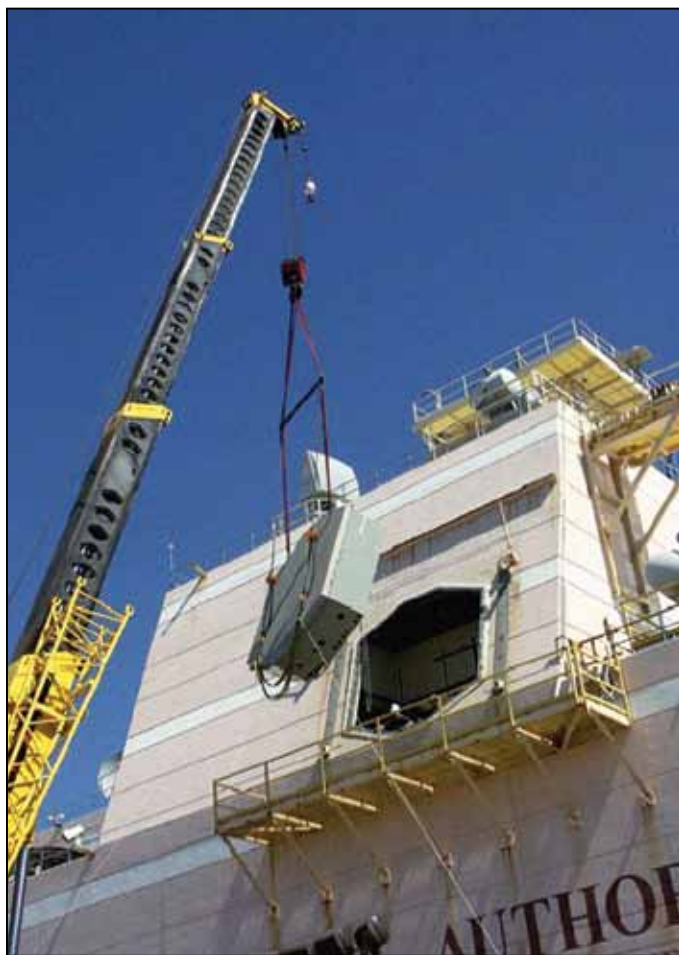
Figure 5. SPY-1A Array Being Uninstalled from the SWEF
