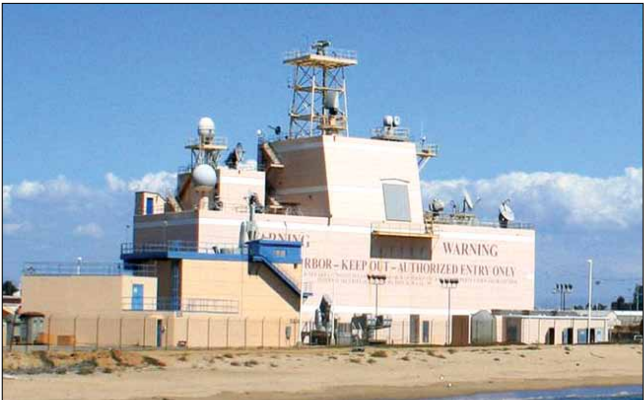
Figure 8. SWEF with the VSR Installed
